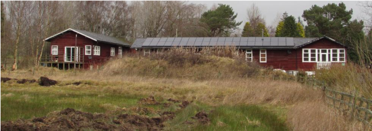
Fig. 4 View facing north towards application site showing former spoil heap
