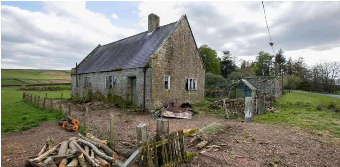
Plate 1. View of the north and eastern elevations. Note the existing boundary fencing, the large verge, the gateposts to be repositioned, and the timber shed.
