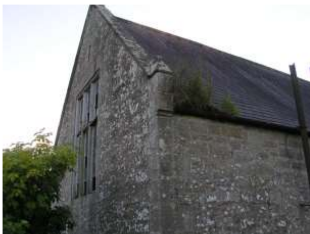
South gable from the southeast
