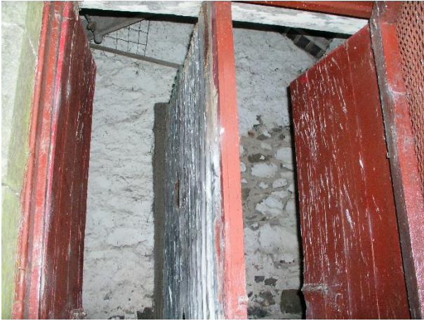
Upper floor of Building 3.
