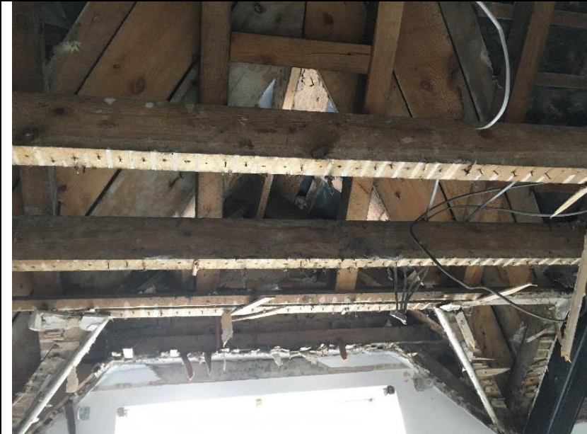
11. Internal attic viewed from stairwell
