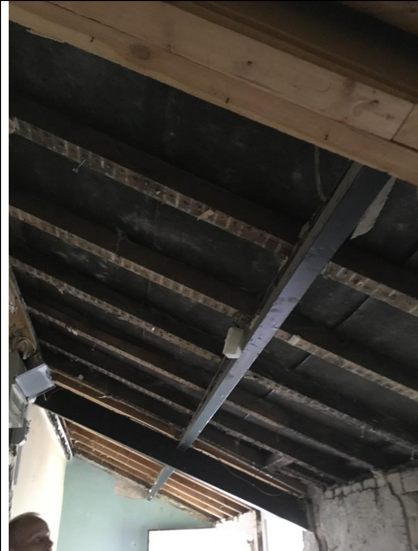
9. Internal, single storey kitchen
