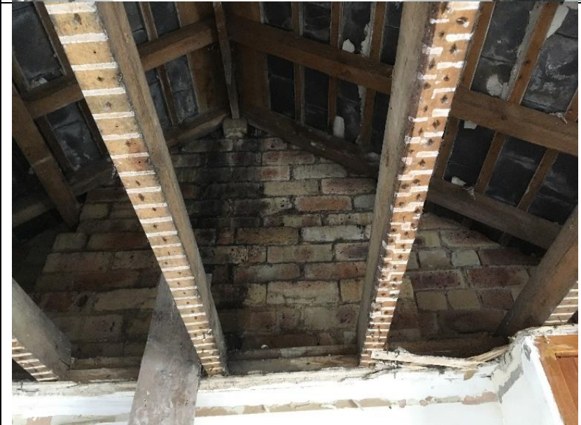
12. Internal attic viewed from second floor bedroom
