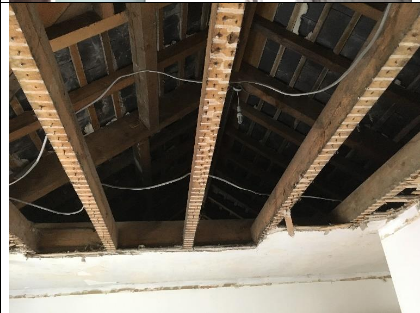
10. Internal attic viewed from second floor bedroom
