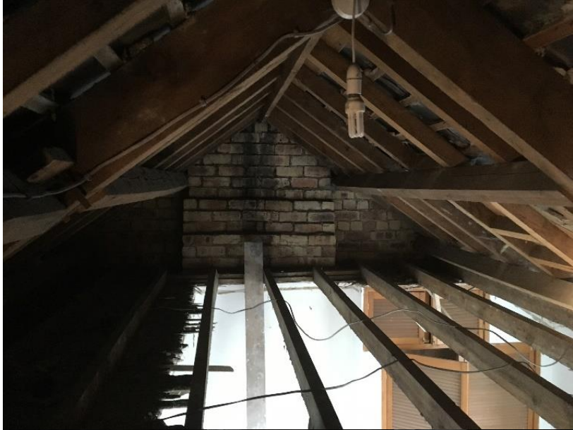
13. Internal attic (north) viewed from loft hatch
