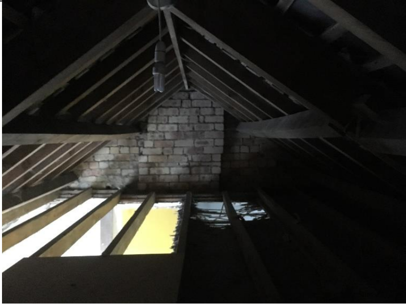
14. Internal attic (south) viewed from loft hatch
