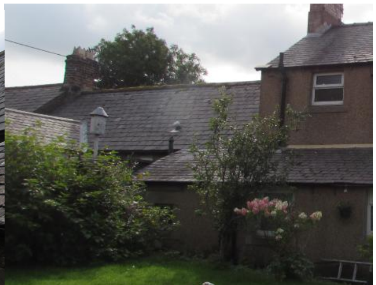
Rear elevation of properties showing overlapping single storey element
