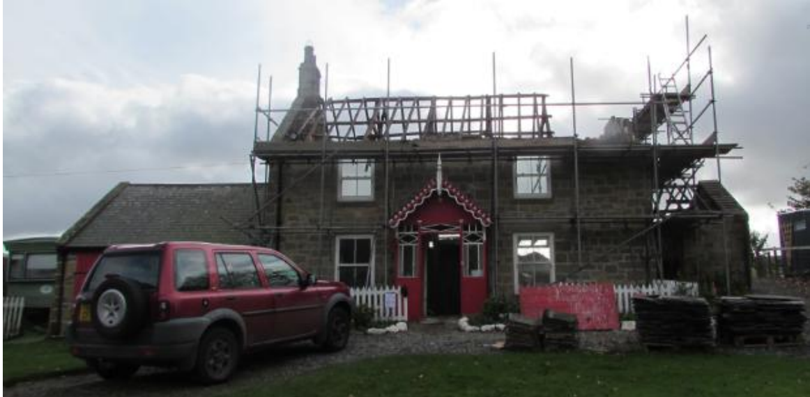
Photograph taken during site visit on 12.10.2017 showing ongoing works
