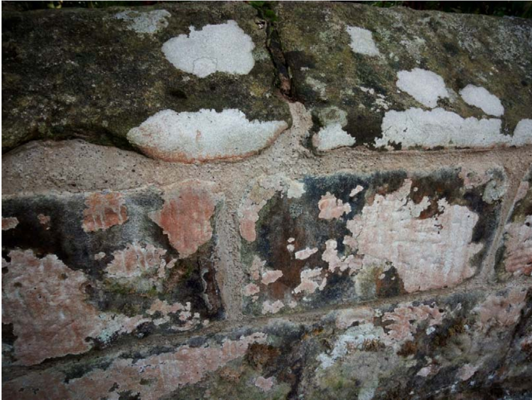
Photograph 2 – Mortar Sample in Parapet
