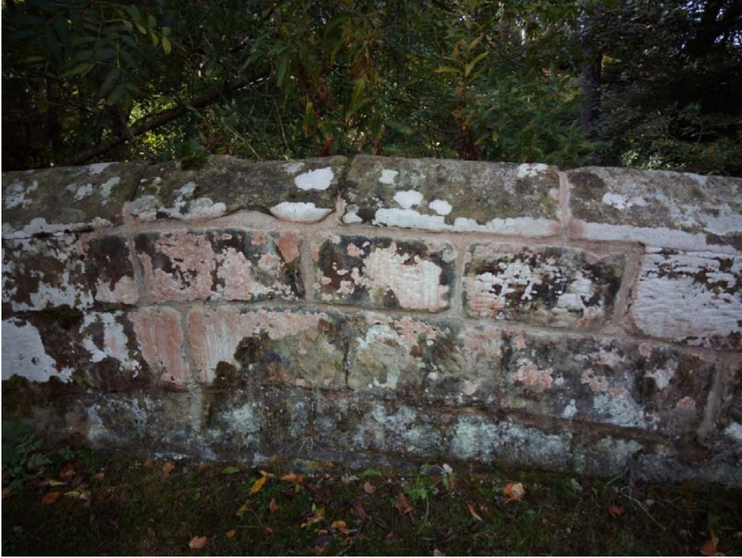
Photograph 4 – Mortar Sample Panel in Parapet.
