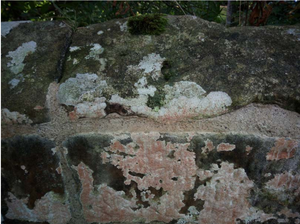
Photograph 3 – Mortar Sample in Parapet
