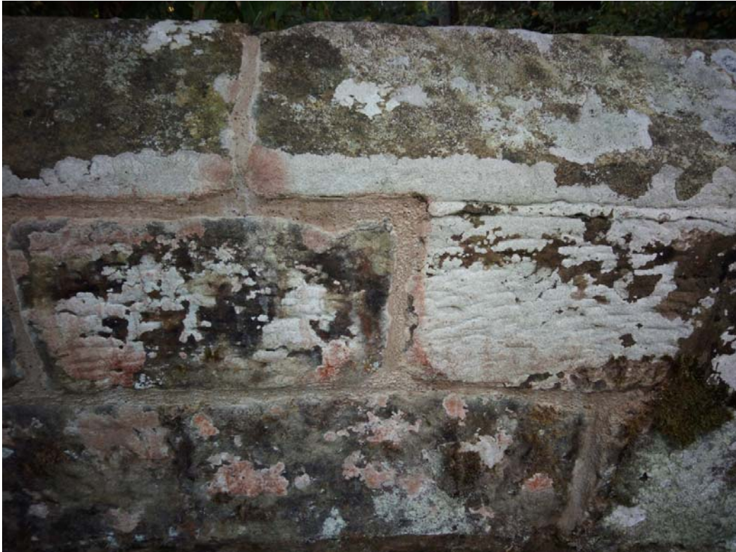
Photograph 1 – Mortar Sample in Parapet Masonry
