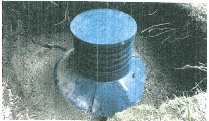
Turret invert extension during installation
