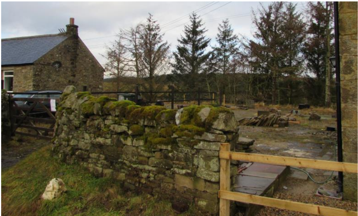
View facing towards application site from adjacent road; existing vehicular entrance visible to left
