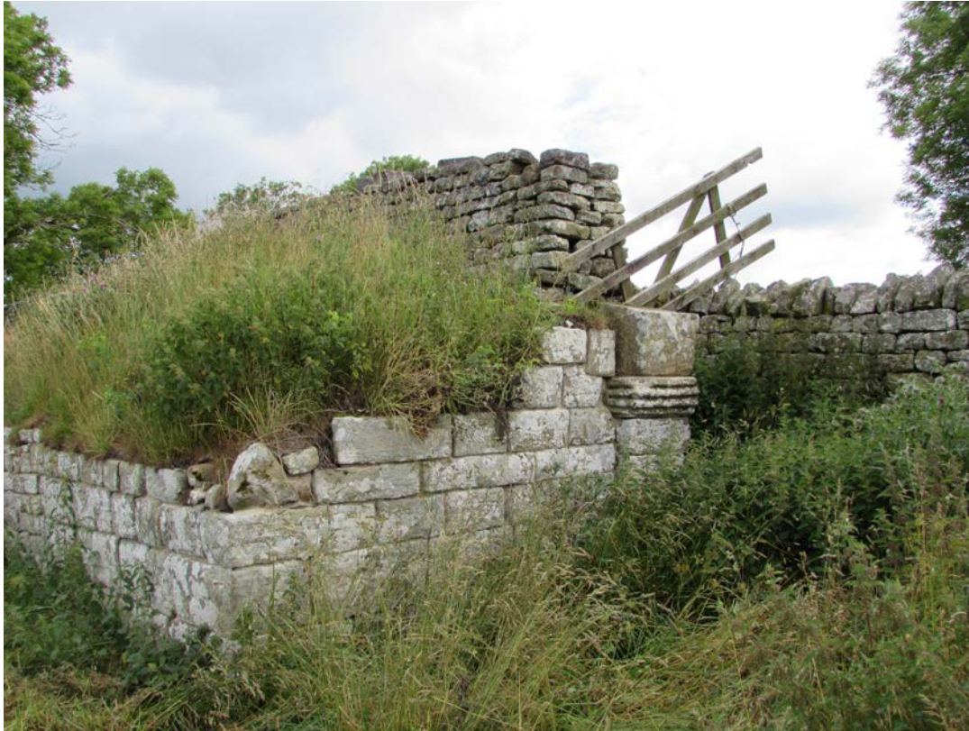
Figure 2: looking east, towards fort from outside of its boundary
