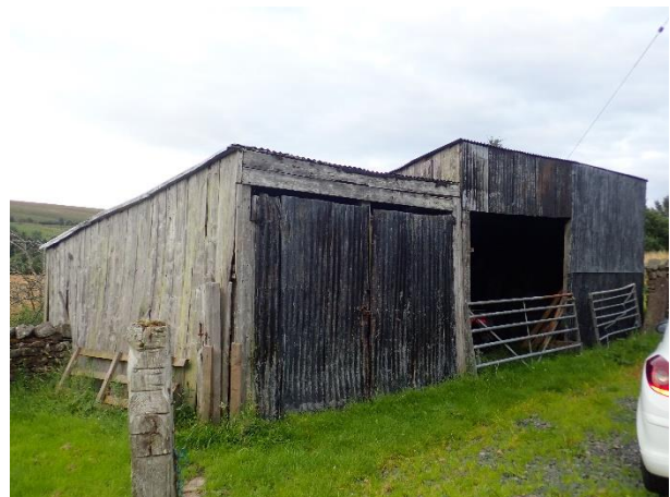
Building 3 from the southwest
