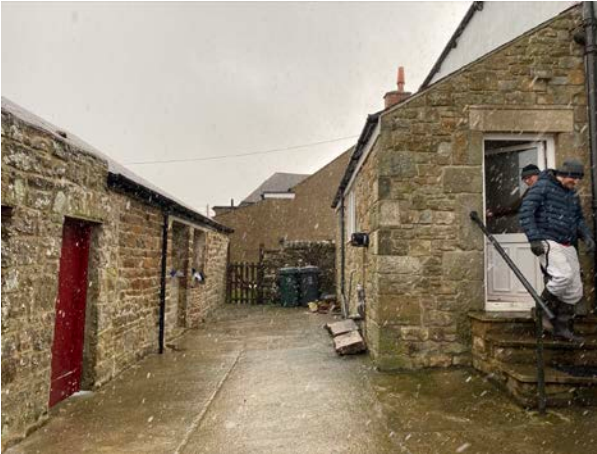
Fig 7 Field house kitchen to right, barn to left
