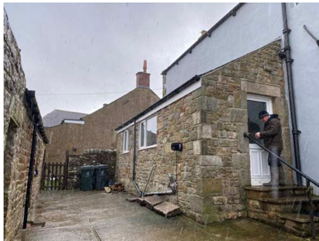
Fig 13 raised ground floor of Field House kitchen
