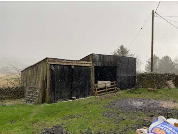
Fig 9 timber barns to be demolished
