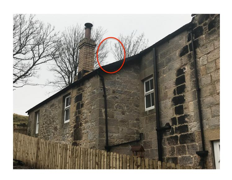
Install woodburner flue to heat pub's upstairs living accommodation. The flue will be installed behind the existing chimney, 1.5m from the hole in the roof. It will be a black flue with cap, very similar to the one shown.
