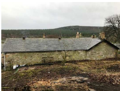
Existing garden level at rear elevation
