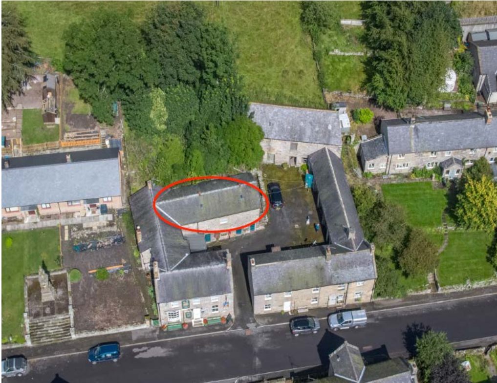
Fig 11 solar panel location
