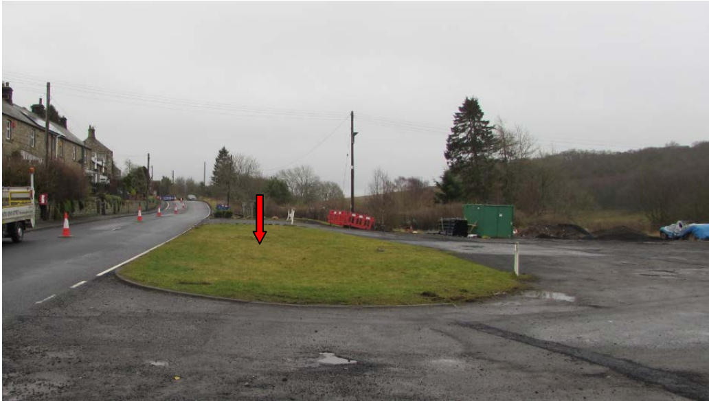
Figure 3: View of application site and A68 from the north-west
