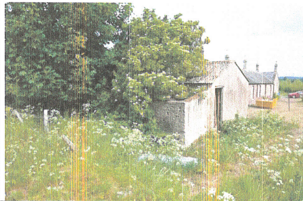
Photograph 3: Southern elevation of outbuilding
