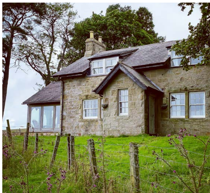
Fig 1. Existing photo of cottage
