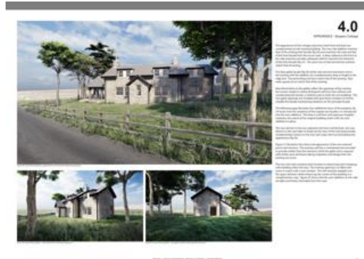
The Cottage (extension shown to left)
