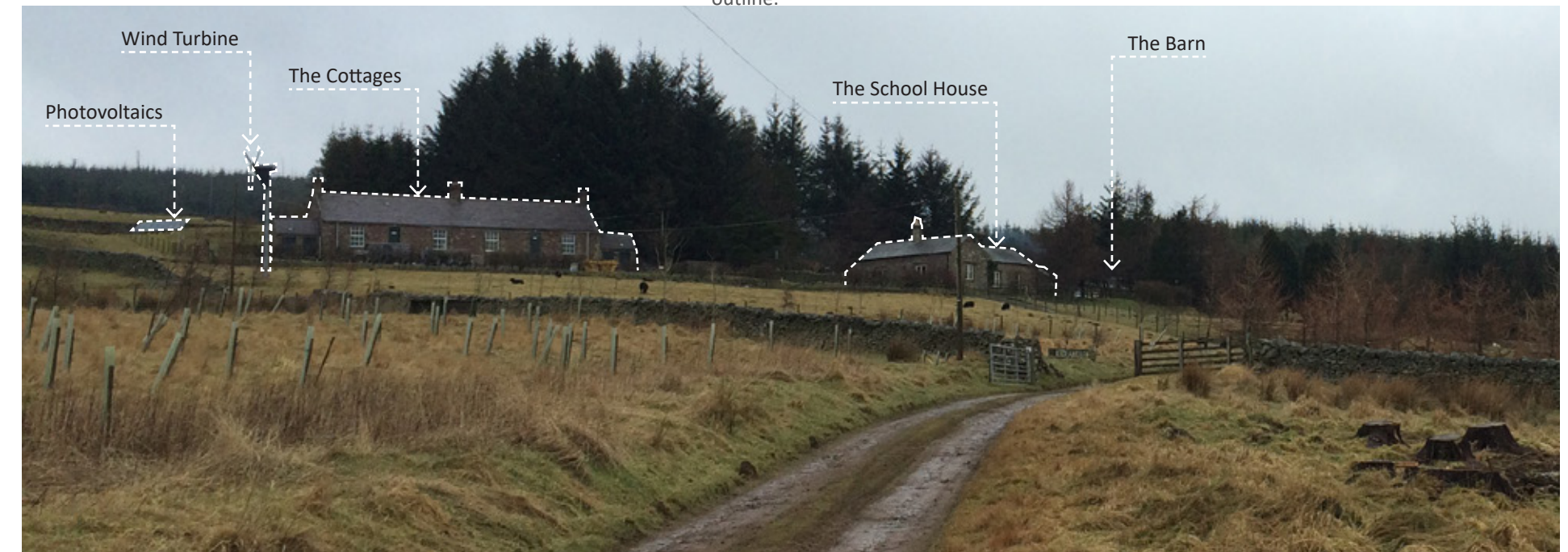
Fig.05 _ View of existing site on arrival depicting existing buildings which have since been restored.
