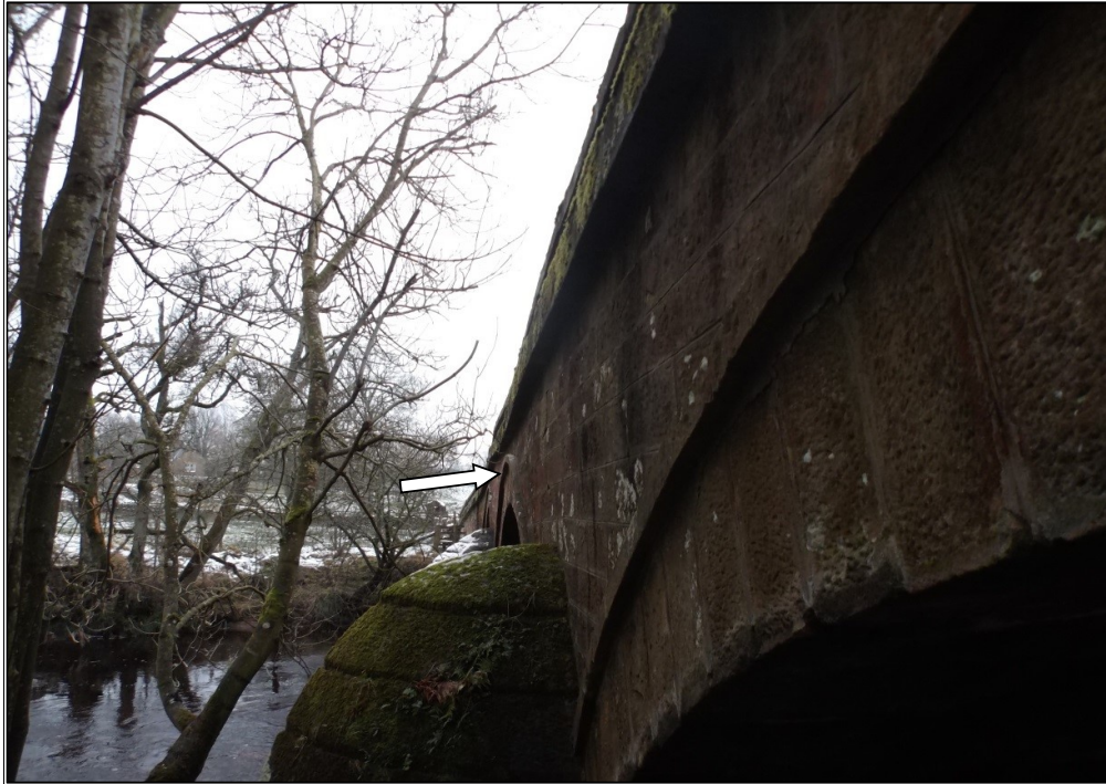
Photograph 3 – Bulging spandrel wall above west pier upstream elevation
