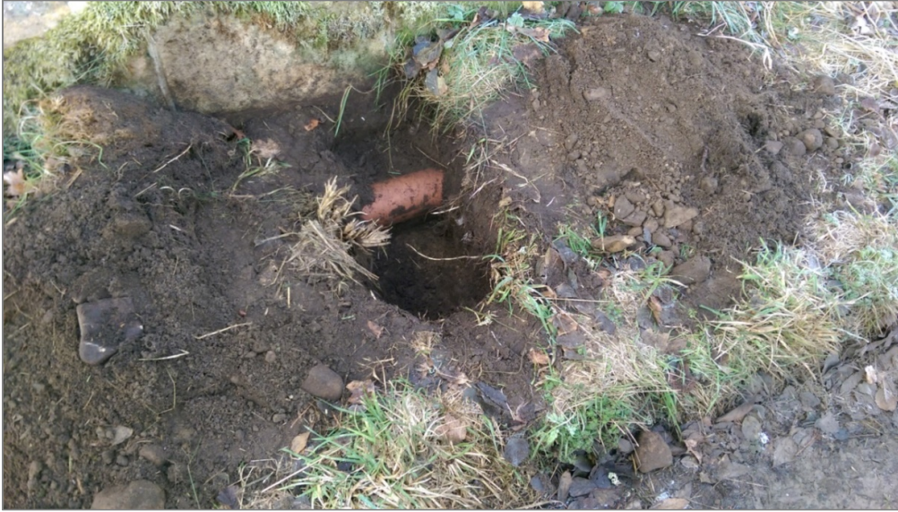
Photograph 10 – Downstream verge BT duct (05/12/2016).
