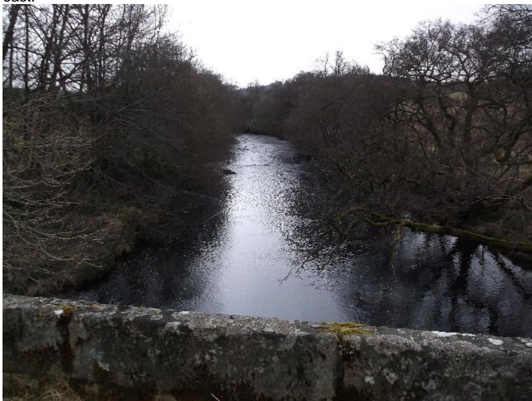
Photograph 5 Overview of Tarsset Burn and broad-leaved woodland, looking north east.
