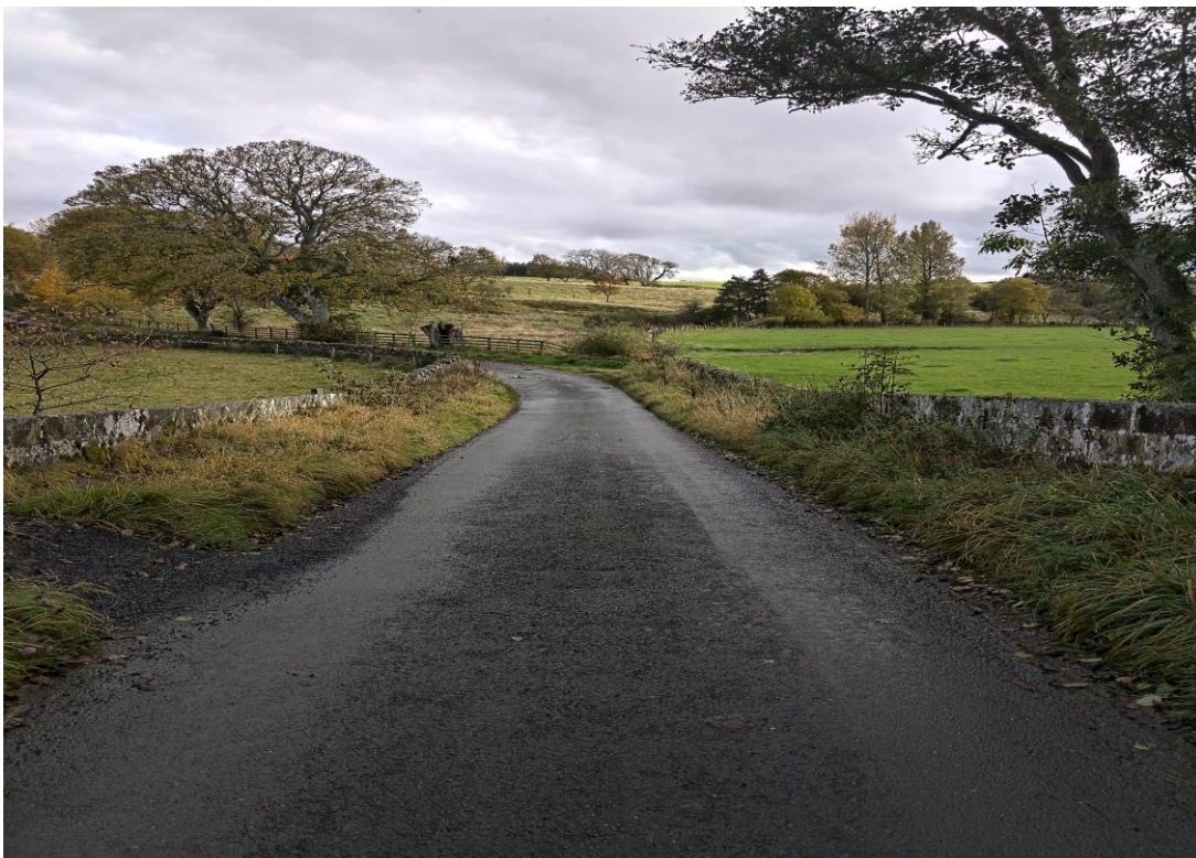
Figure 4: Vegetation growth on the verge of bridge
