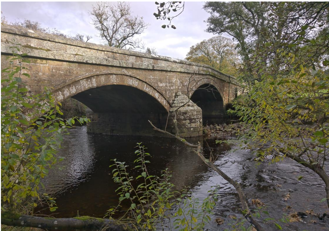
Figure 3: Redmire Bridge considered from the south
