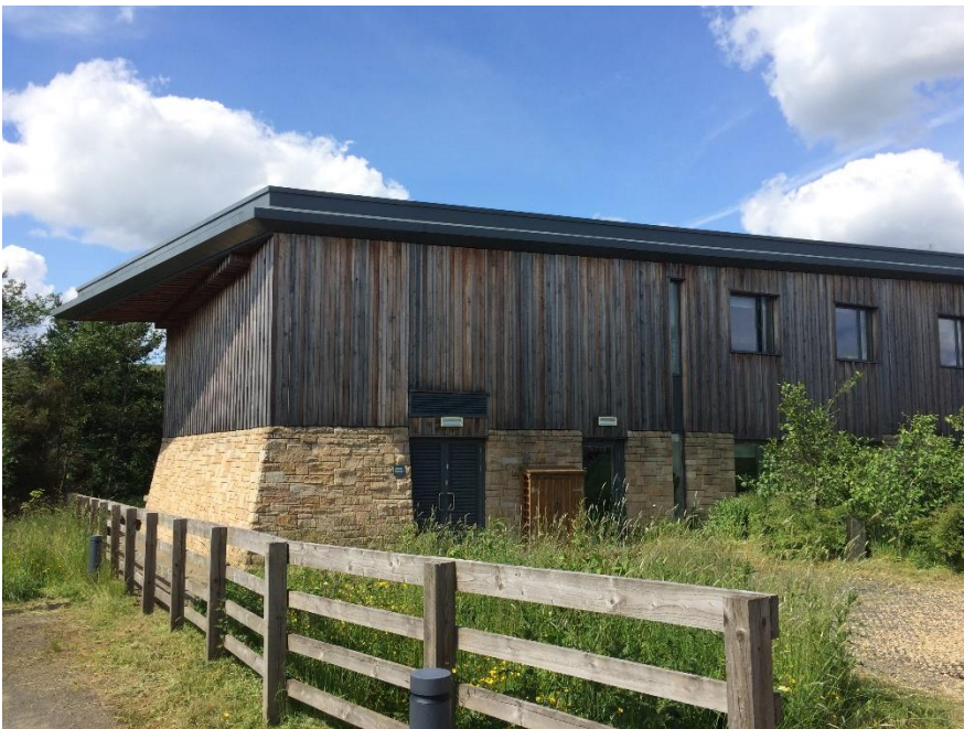
Photo 2 – untreated larch cladding and dark grey aluminium fascia and glazing of the Sill provide contemporary design cues employed in the planetarium.
