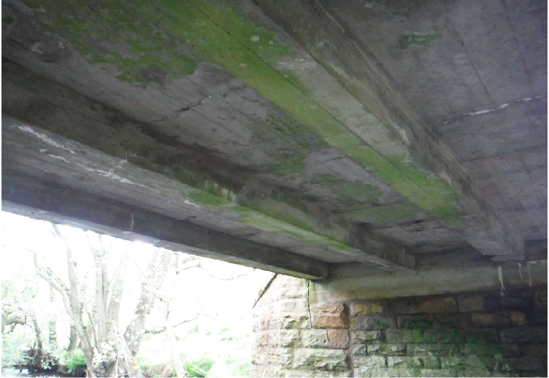
Photo 5 Underside of deck.
