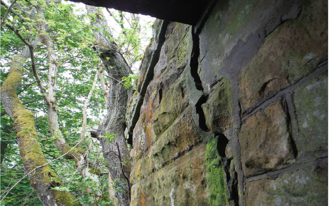
Rotation at top of south abutment
