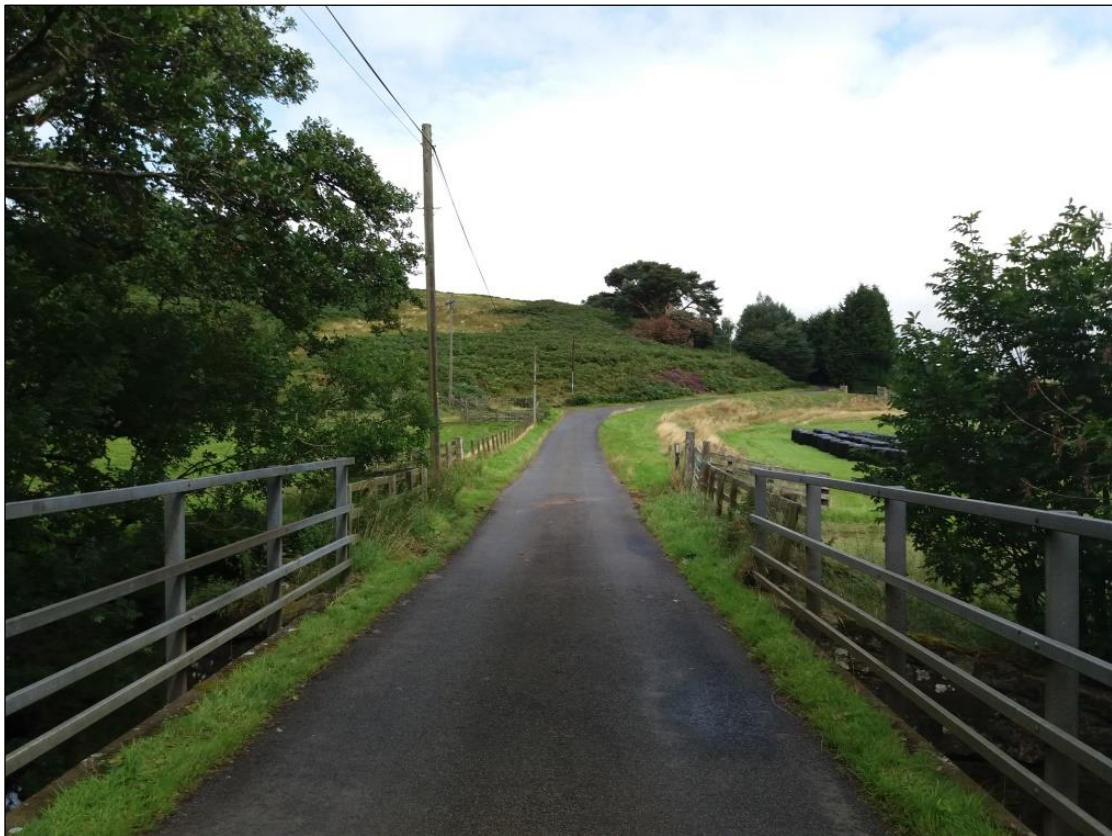
Figure 3 - View over structure (looking north)
