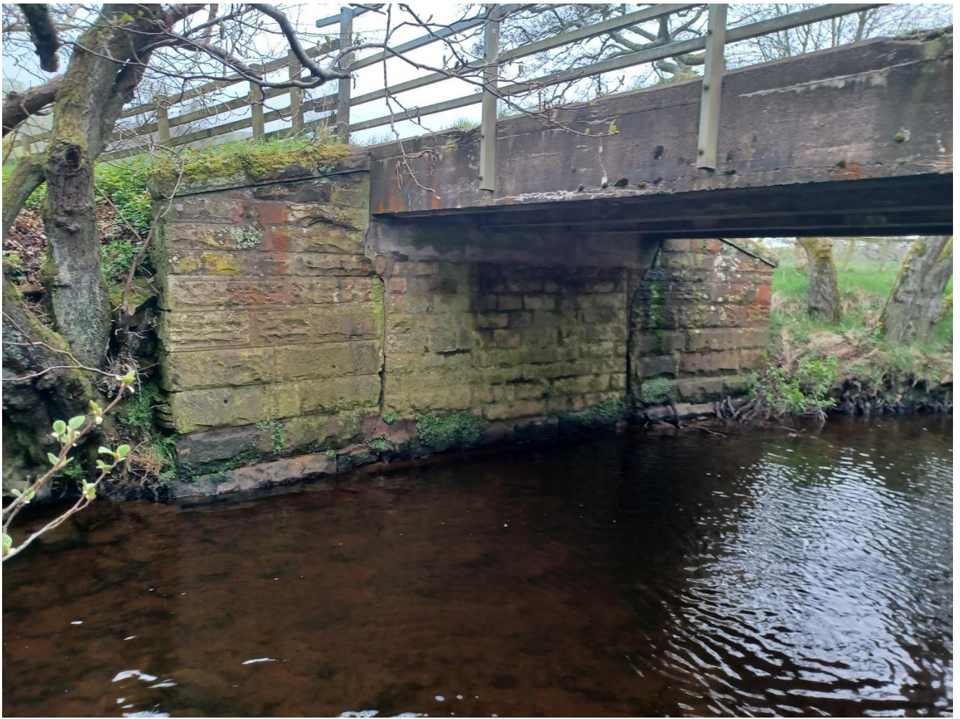
Figure 11 view of underside of bridge from downstream
