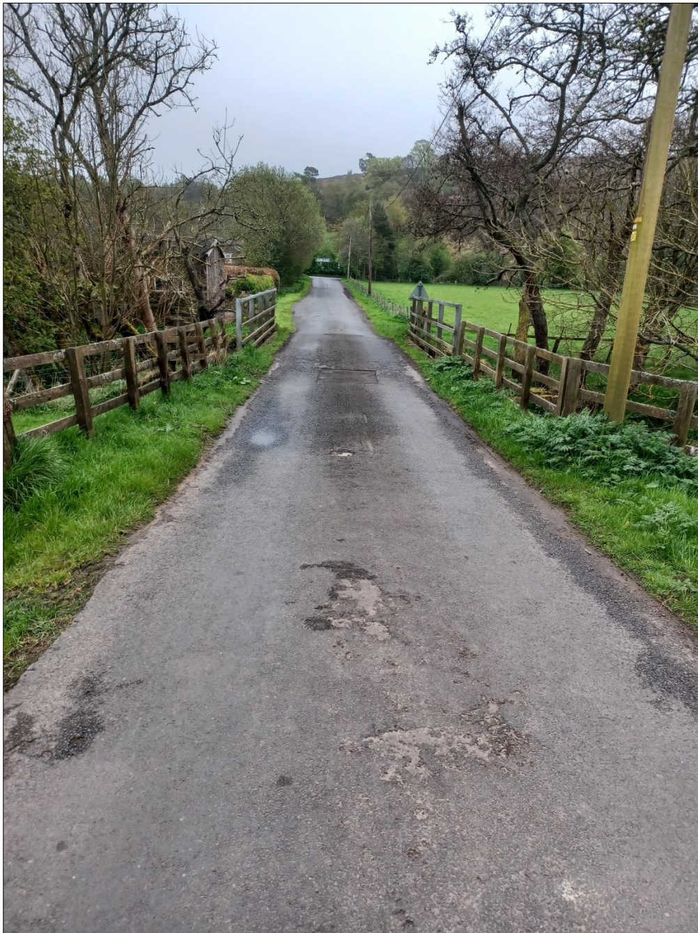
Figure 5. Northern approach to bridge
