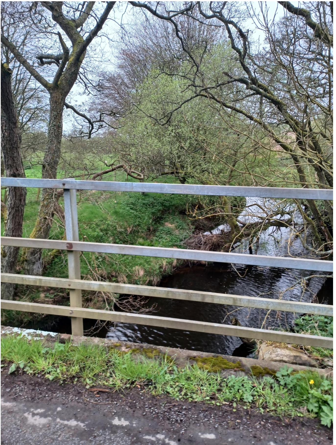
Figure 7. bridge deck looking upstream
