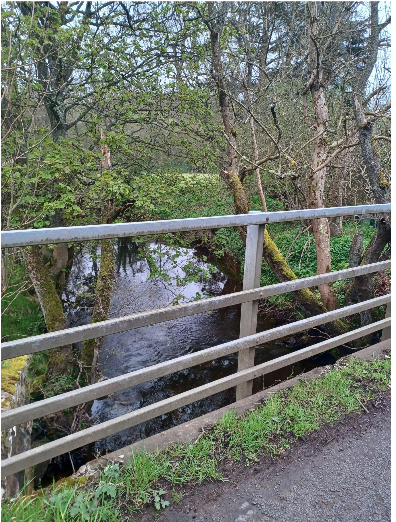
Figure 6. bridge deck looking downstream.
