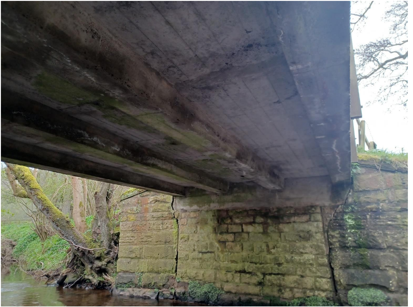
Figure 9. underside of bridge deck
