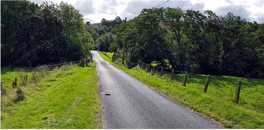
Photograph 1 – Swindon Kennels Bridge as on 28 th August 2019.
