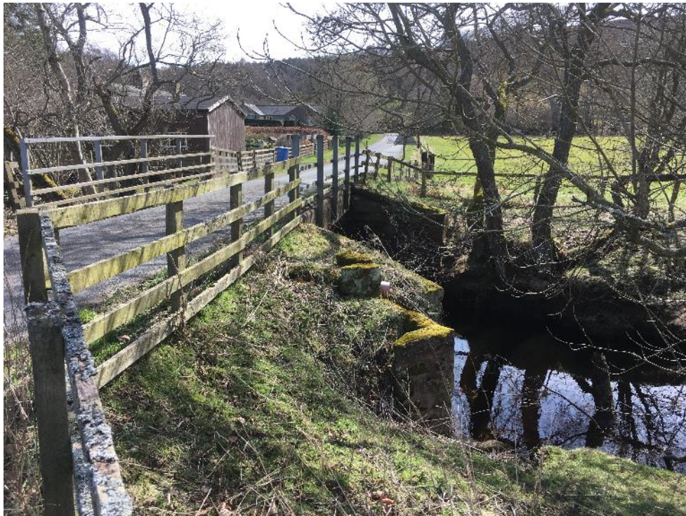
Photograph 3 View of the bridge and habitats to the south, including Harehaugh Farm buildings.
