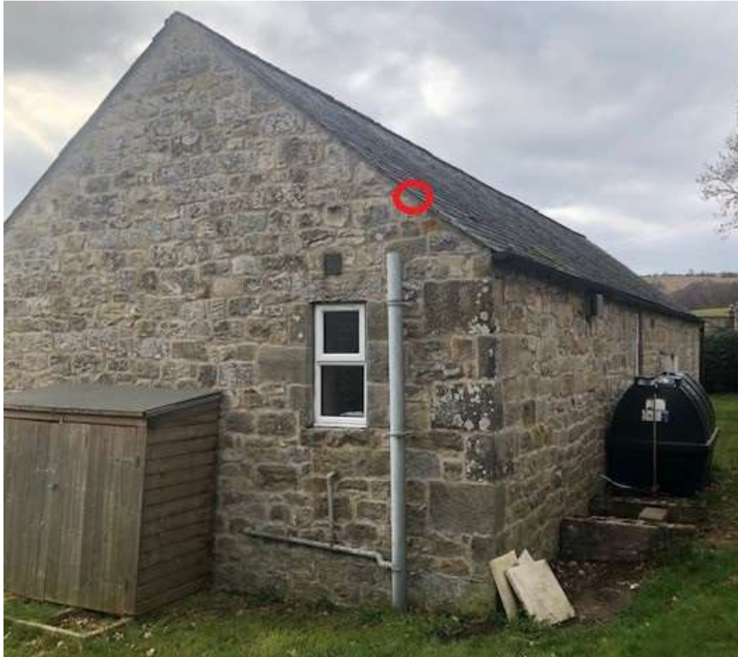
Photograph 11 – Building reference A, northern gable end with bat re-entry location circled.
