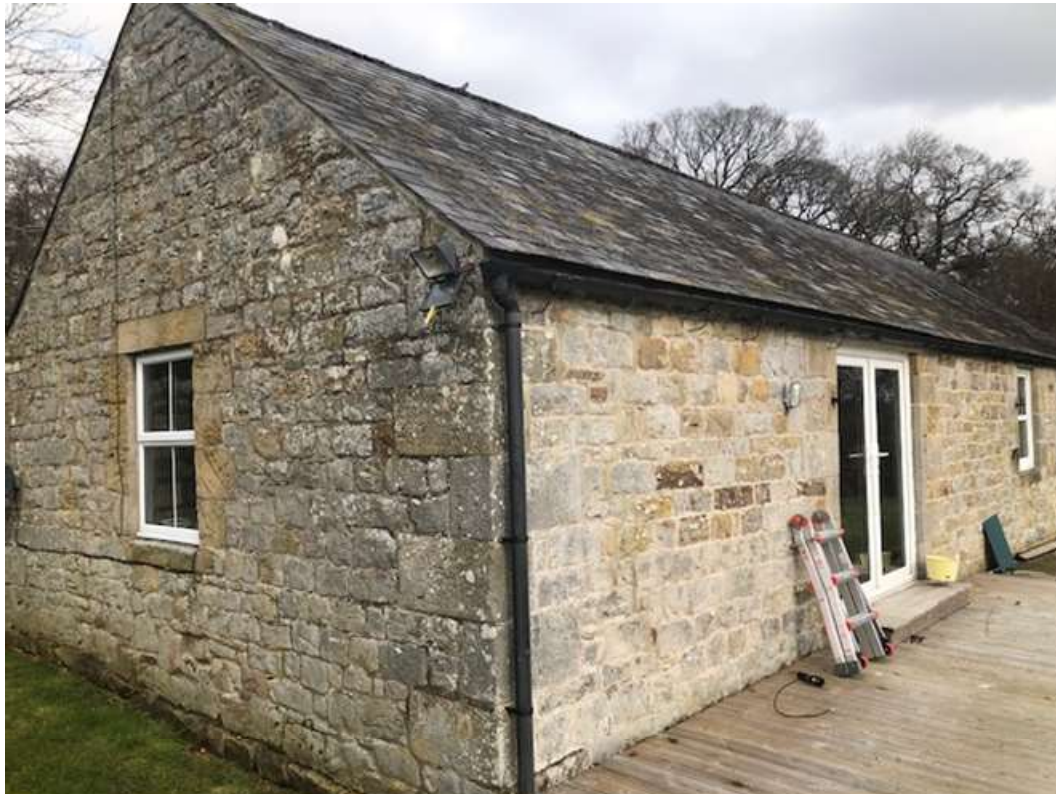
Photograph 1 – Building reference A, southern gable end and eastern elevation.
