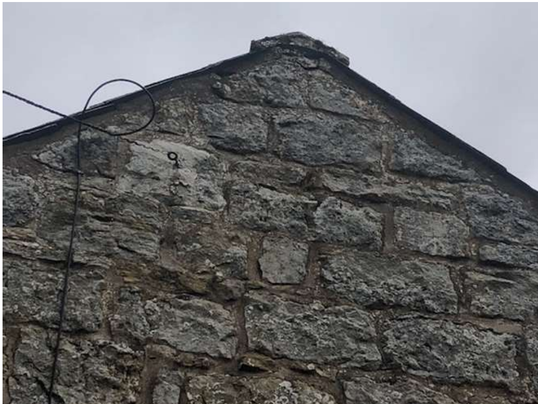
Photograph 8 – Building reference A, southern elevation gable end features.
