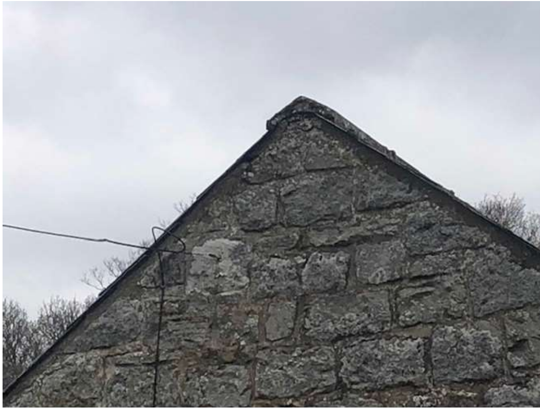
Photograph 7 – Building reference A, southern elevation gable end.
