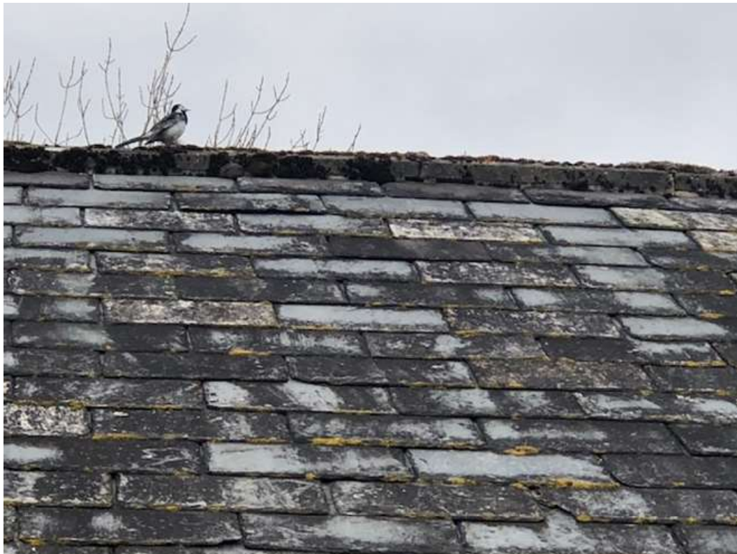
Photograph 10 – Building reference A, western facing roof features.
