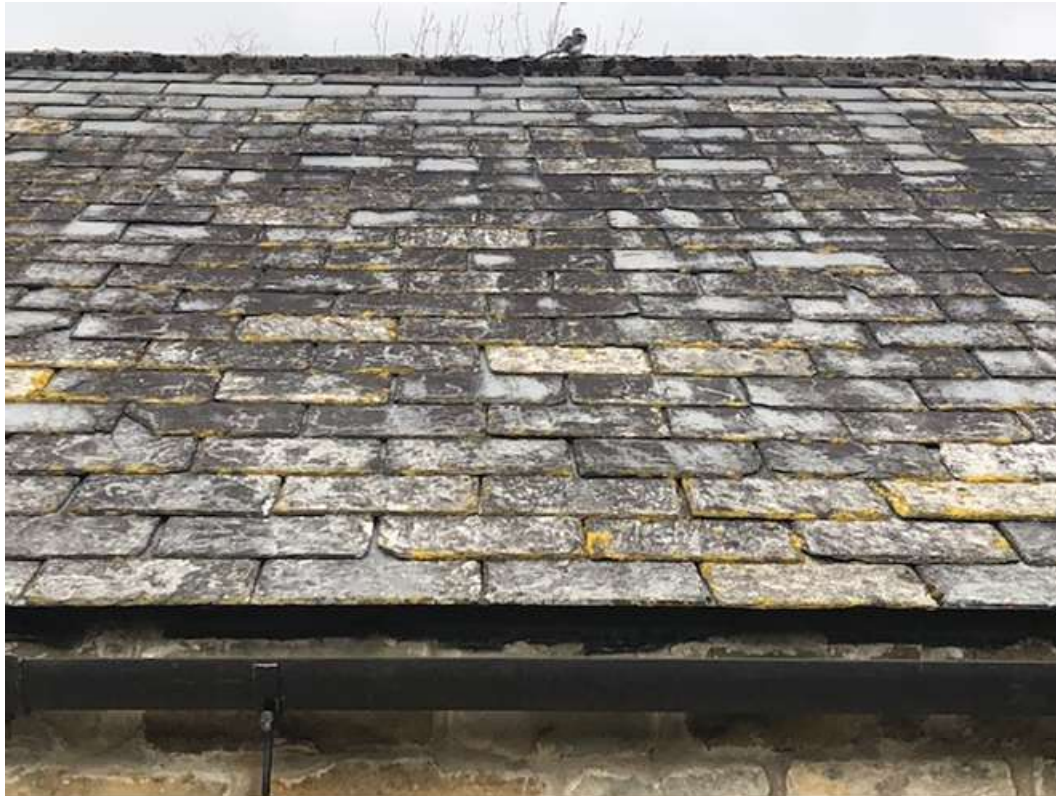
Photograph 9 – Building reference A, western facing roof.
