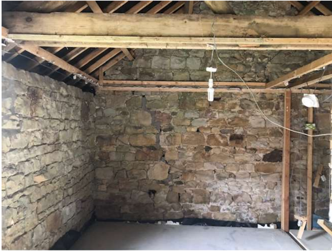
Photograph 5 – Building reference A, south face of interior dividing wall.
