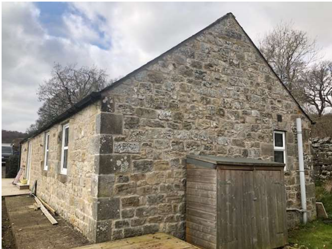
Photograph 2 – Building reference A, northern gable end and eastern elevation.
