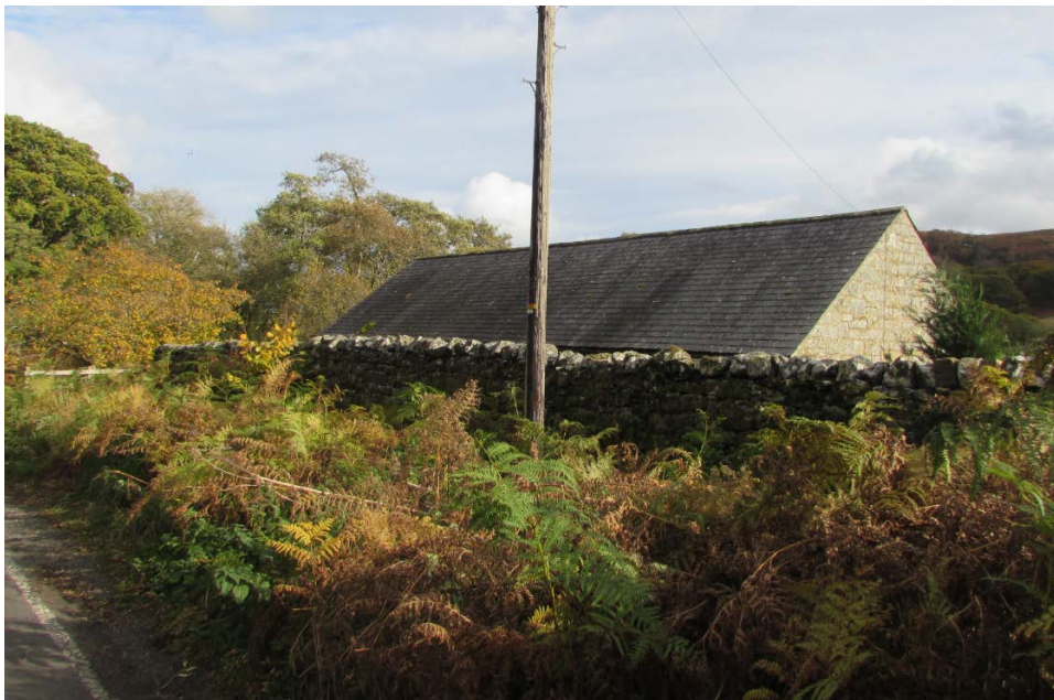
Figure 3: View to the rear of the property from the road
