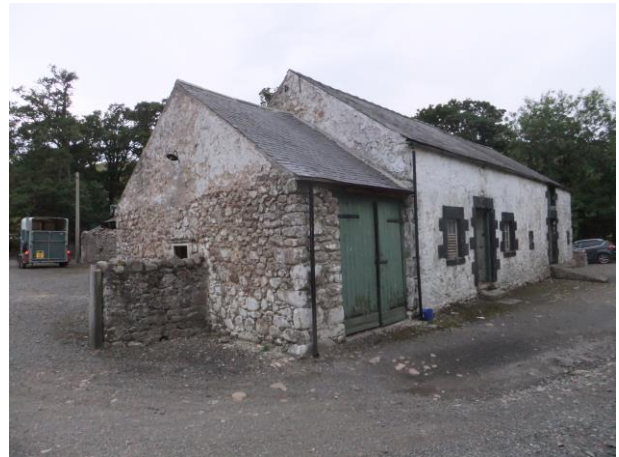
Generator room and southeast wing viewed from the north.
