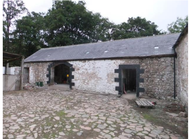
Southeast wing of the barn viewed from the south.
