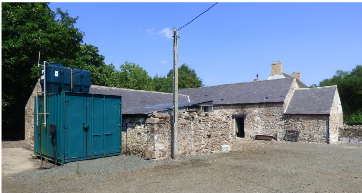
The group from the south-west – Southern Yard Wall, incorporating remnant of former kennels, in centre
