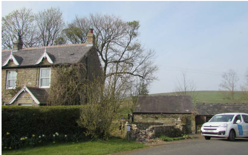
Figure 3: Site showing existing buildings located towards the highway
