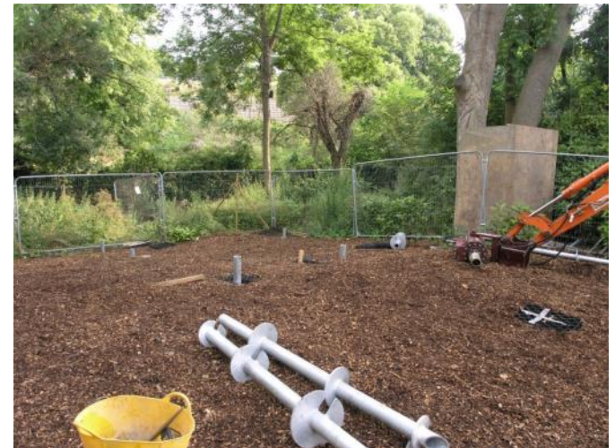
Screw piles being used in sensitive areas near trees
