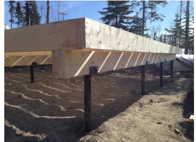
Timber base on screw piles
