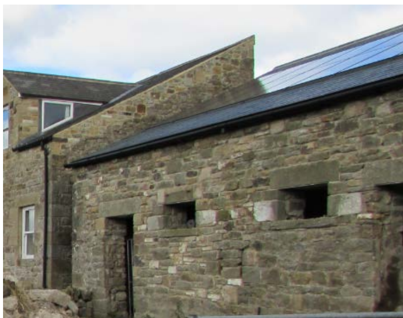
Figure 6: Solar panels to the roof of Unit 1.
