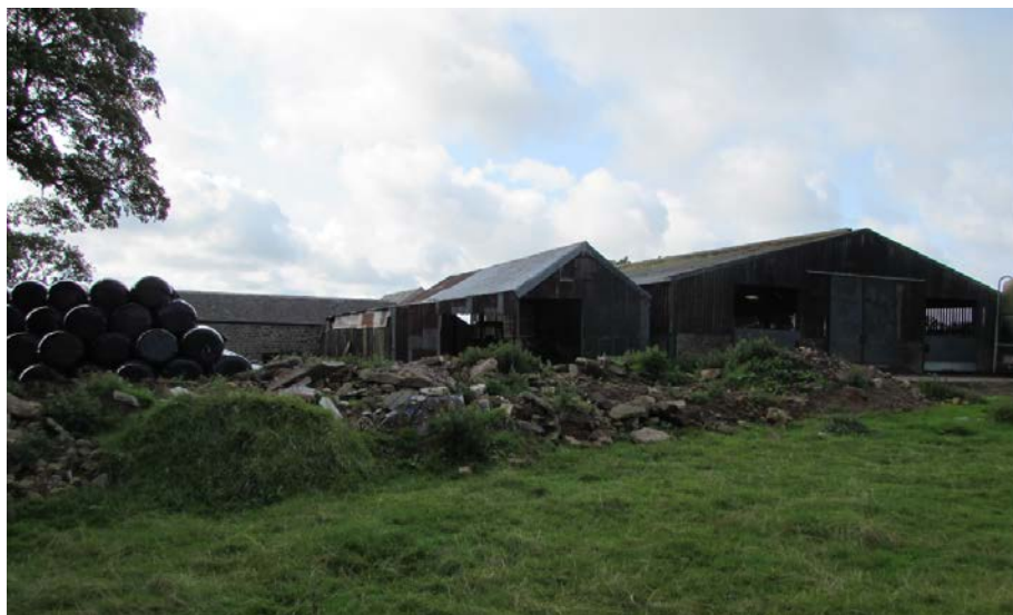
Figure 2: View towards the proposed location of the building from the east
