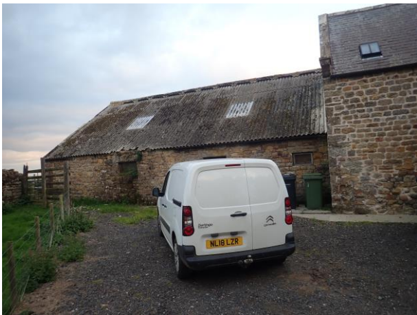
The barn viewed from the north.
