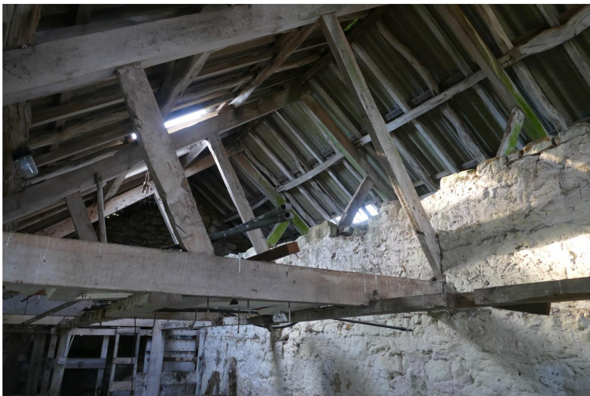
Roof Structure, looking North-West
