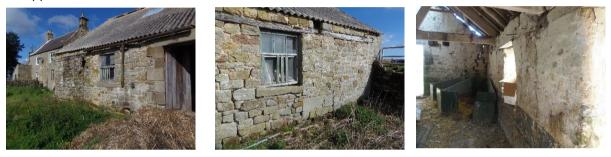
Generally speaking, we are satisfied that the repairs you have scheduled, along with further consideration of drainage and possibly some external paving to the southern side to control water runoff, are the minimum necessary in order to restore the building to a structurally sound and weathertight condition.
