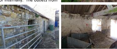
There are a number of cracks to the walls to the northern side and the eastern gable and you have sensibly proposed repairs to the cracks along with rebuilding of a significant part of the central and southern sections of the gable wall.
