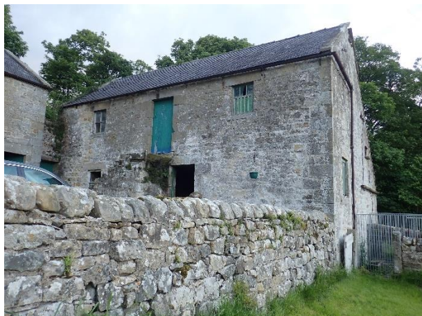
North gable wall
