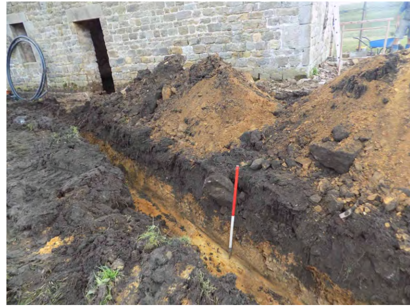
Illus. 09: Trench 1 looking south towards the house
