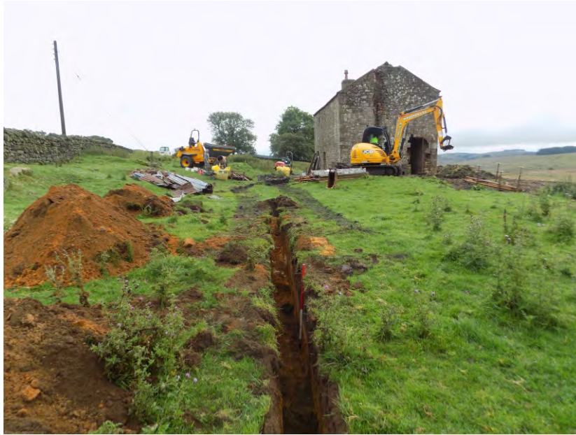
Illus. 08: Trench 1 looking East towards the house
