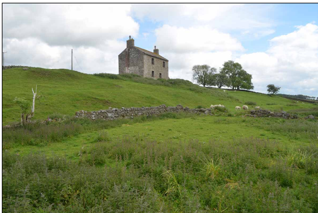
Frontispiece: View from the south-west showing the farmhouse sitting on a prominent position with associated earthworks.
