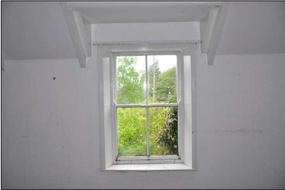
35. Detail of dormer window, rear bedroom, first floor
