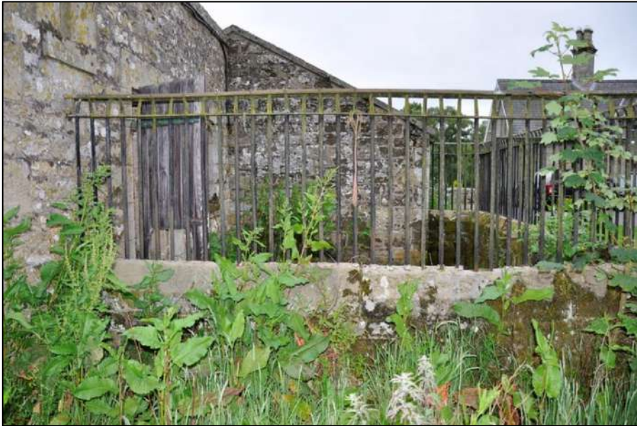
71. Detail of enclosed front yards with railings atop stone walls. Concrete floor surface
