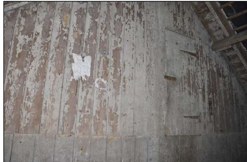
42. First floor timber south-east wall with hay loft opening. Loft floorboards renewed at a lower level (see original level under door)
