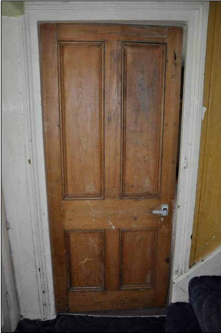
27. Four-panel door in moulded architrave, probably original, to front parlour
