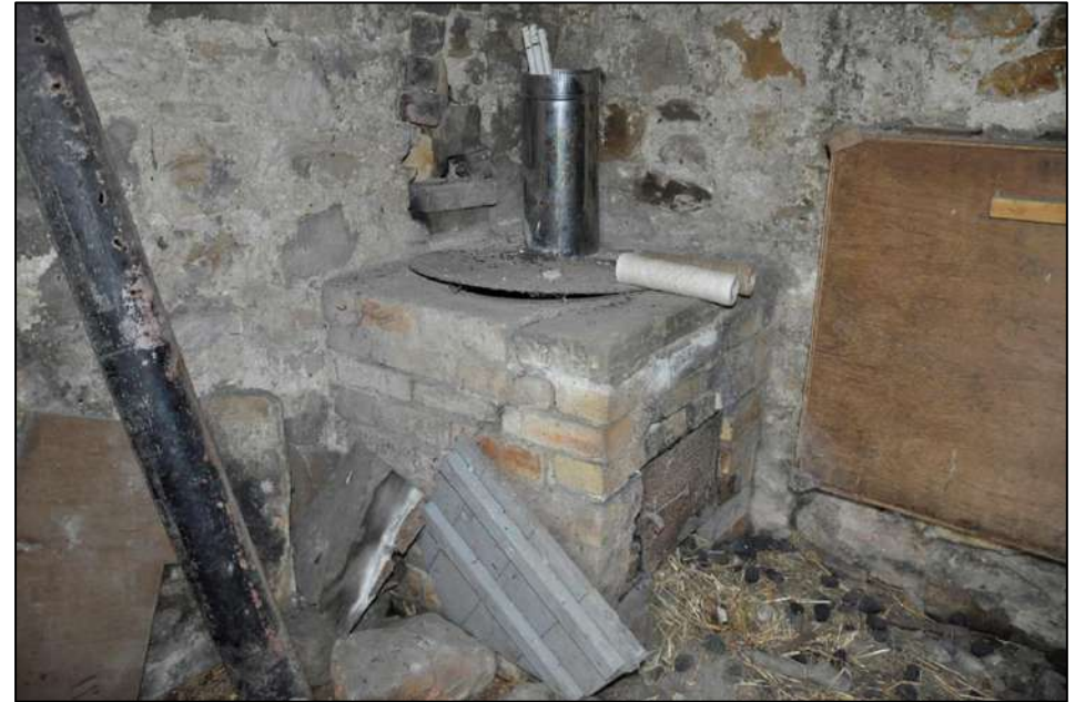
77. Brick copper within boiler house
