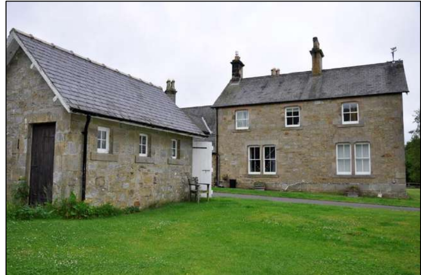
12. Detached outbuilding, looking north towards Evistones House
