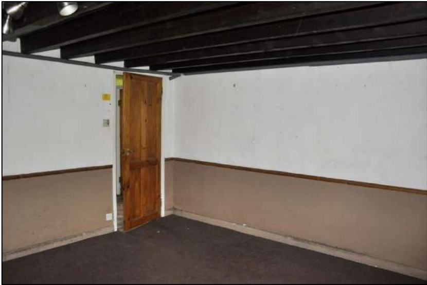
21. Modern four panel timber door to rear parlour
