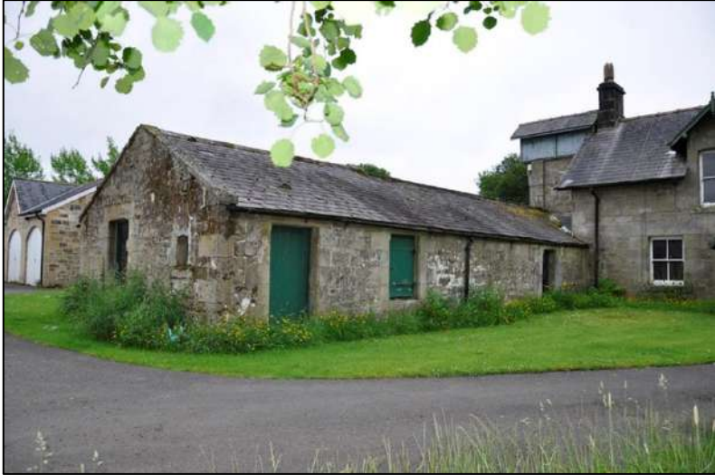
47. North-west elevation of stables, kennels and stores with three openings under a dual pitched slate roof
