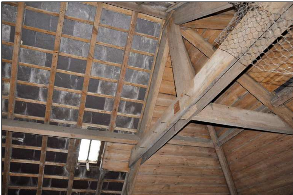
43. King post truss, loft. Much of roof has been renewed
