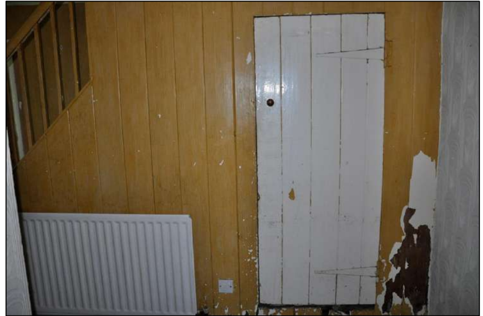
26. Historic, probably original, vertical boarded door with strap hinges set within staircase structure to enclose cupboard within
