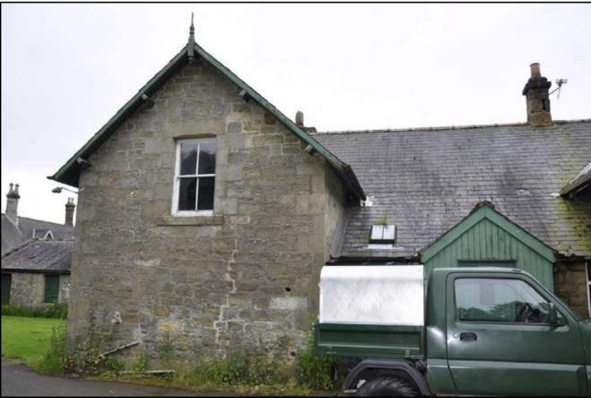
18. North-west gable with one sash window and projecting bargeboards with finial
