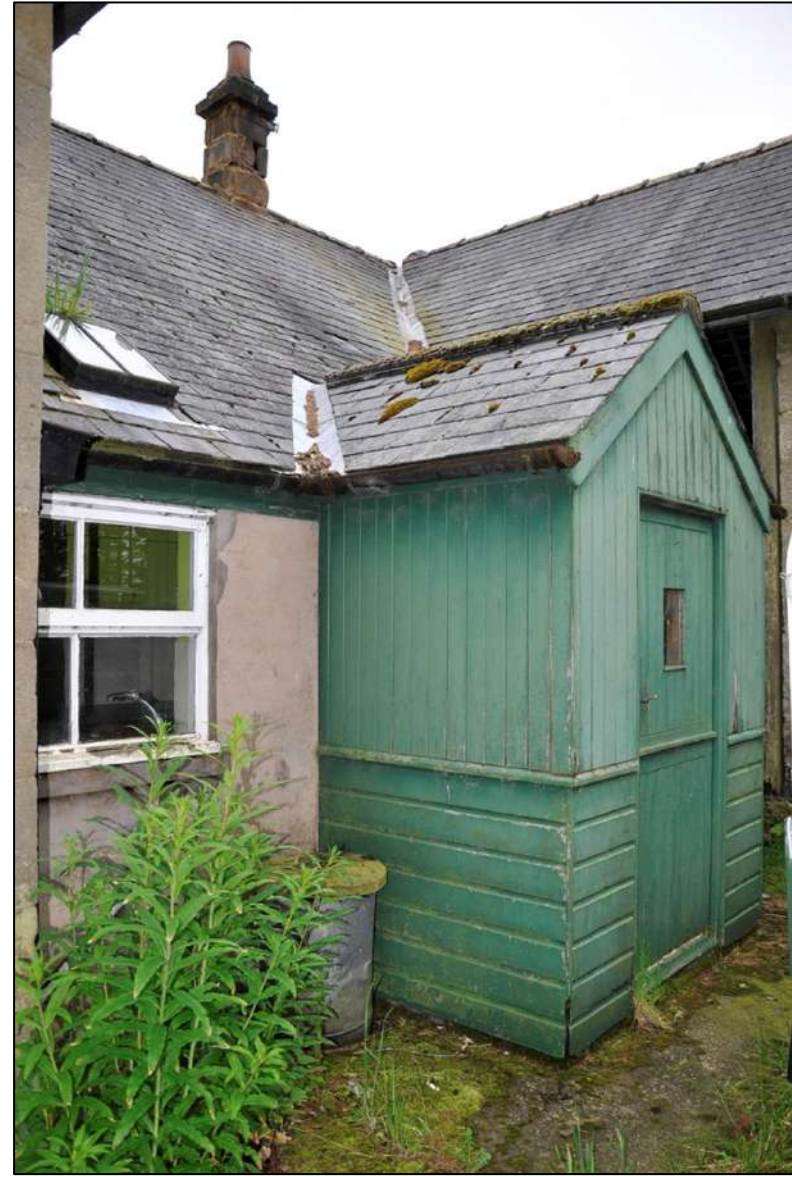
17. Render applied to part of kitchen extension. Stone chimney
