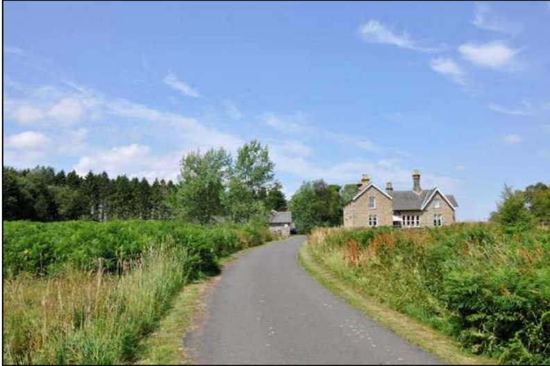
1. Approach to Evistones with Evistones House most prominent in foreground
