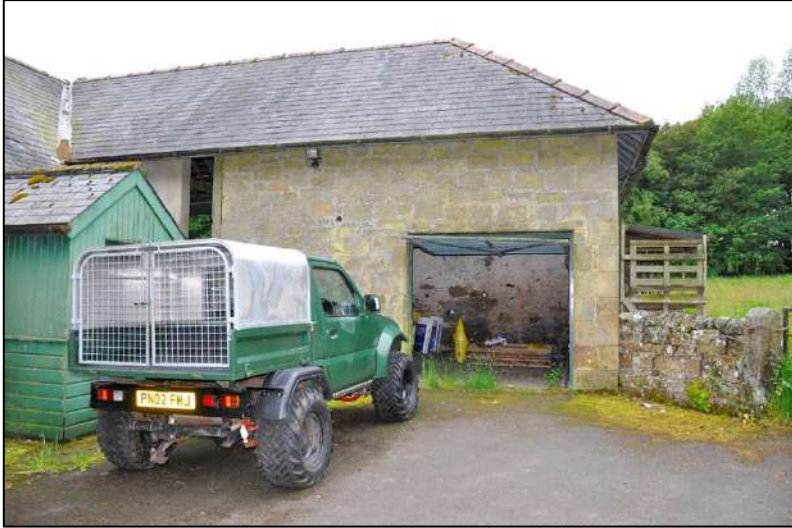
39. North-west elevation to cart shed with wide opening
