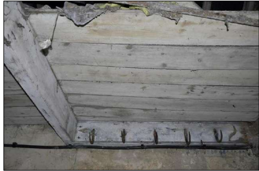
61. Hooks to north-west wall. Note painted wall decoration below
