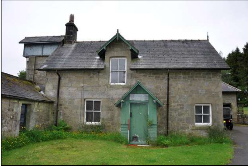
13. North-east front with two over two sash windows, dormer window and later porch (1m x 1m scales)
