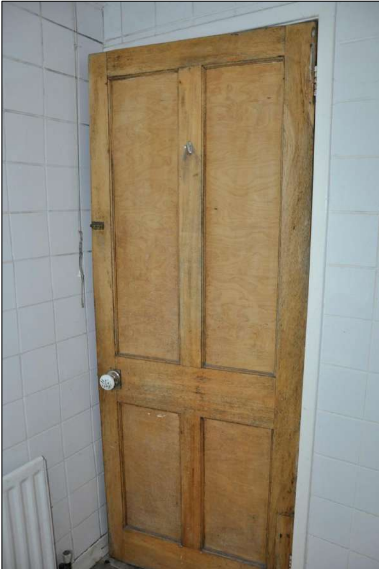
23. Original or early four-panel door to bathroom, resited here when bathroom formed
