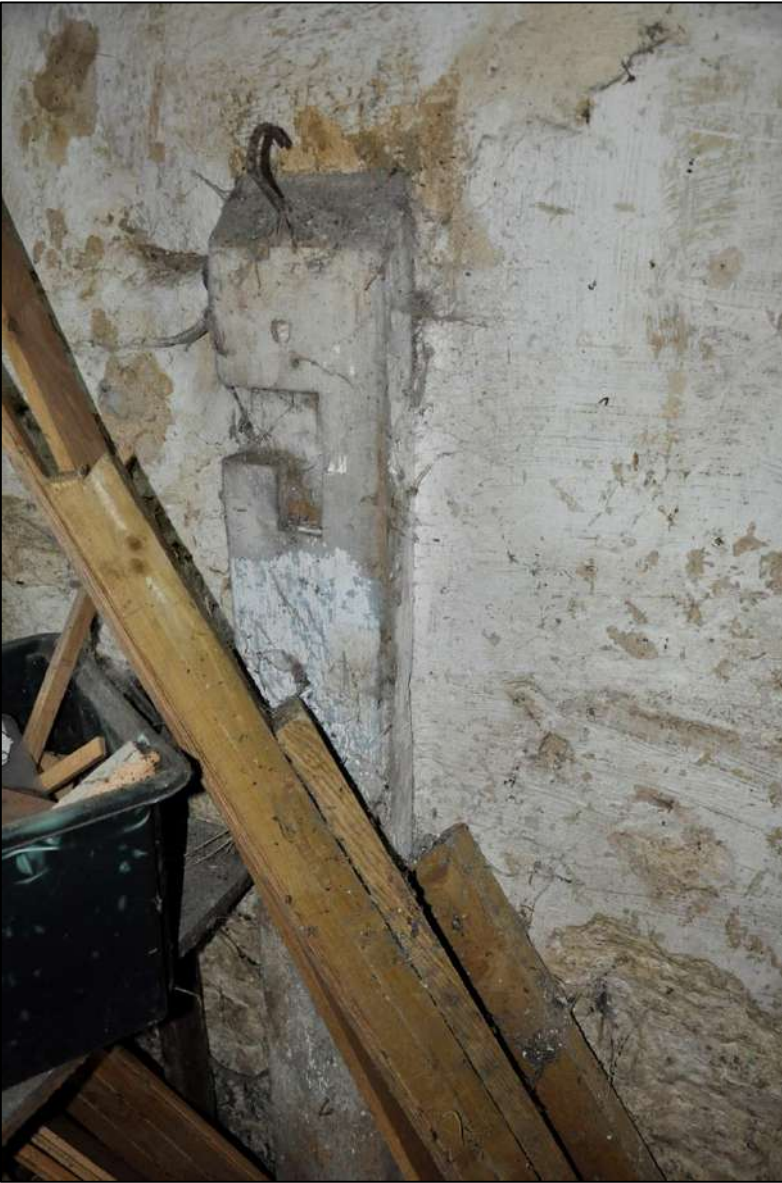
59. Gate post to former stall gate (gate does not survive)
