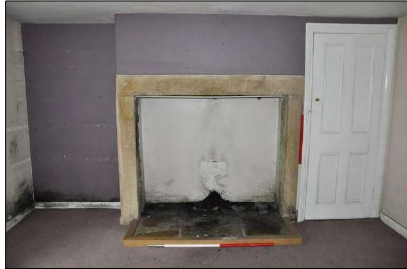
28. Plain stone surround to parlour fireplace (fireplace missing) with adjacent four panel cupboard door with moulded architrave, all likely original components, front parlour
