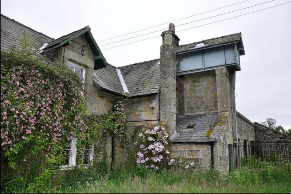
74. Cottage with attached water tank and boiler house
