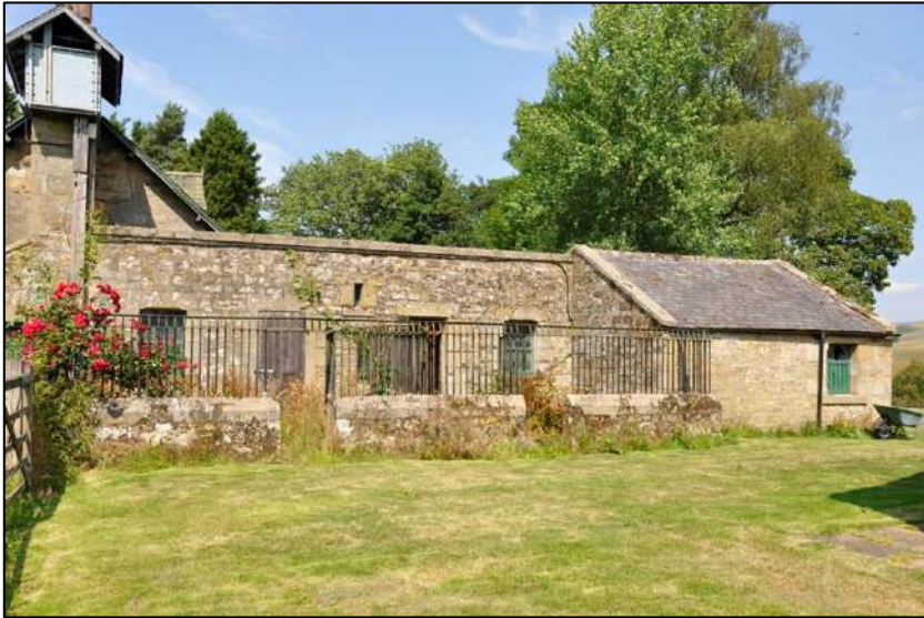
5. Kennels with enclosed yards (centre), stables (right), water tank (left), south elevation
