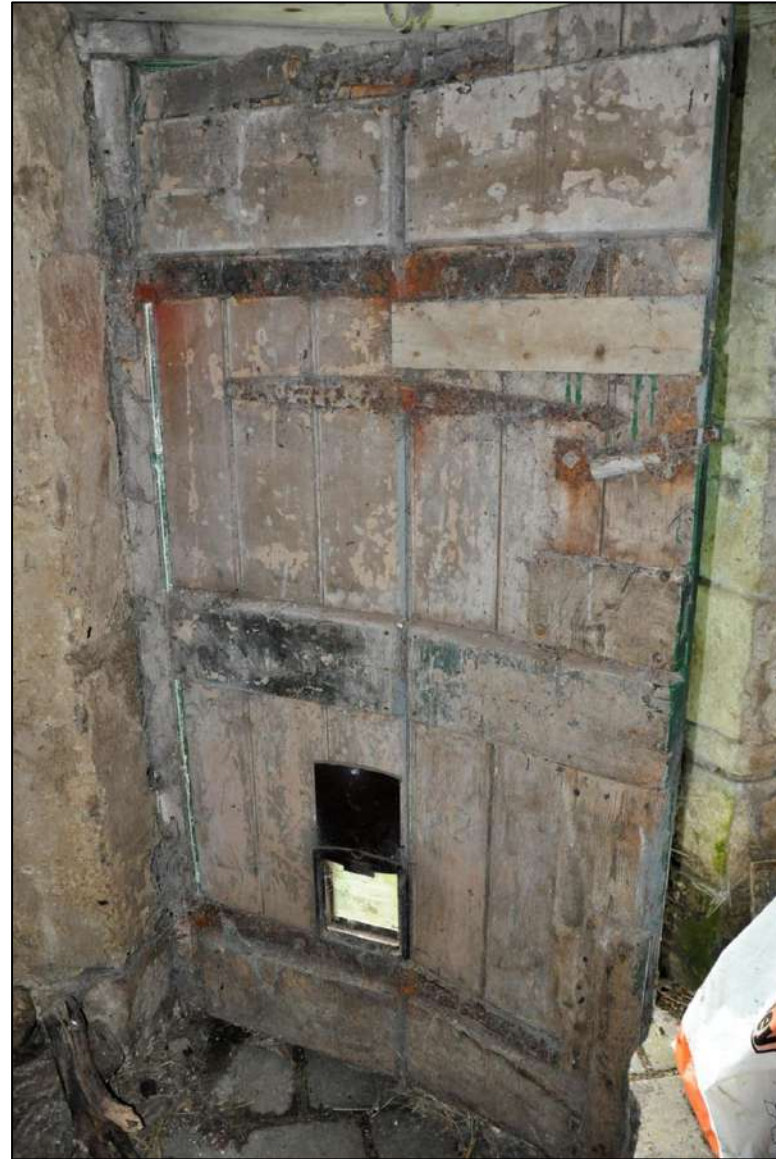
63. Interior view of vertical boarded entrance door
