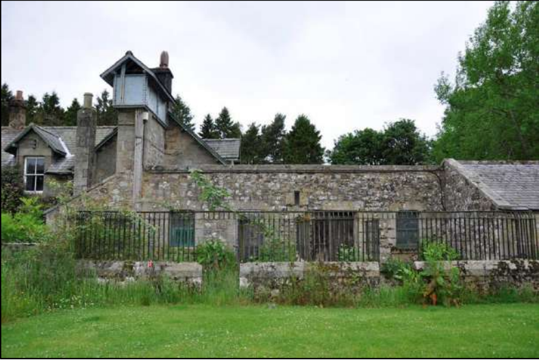
64. South-east elevation of kennels with central dividing store and front yards
