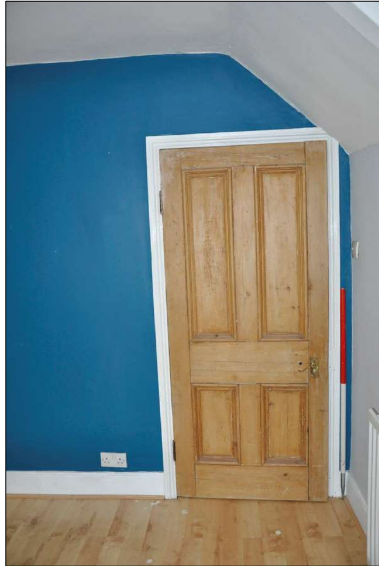
38. Original four-panel door set in moulded architrave, front (western) bedroom
