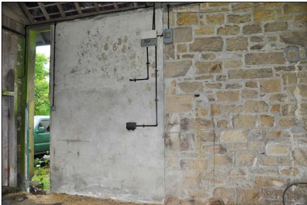
46. Quoins mark south-west elevation of cottage with later kitchen extension (rendered wall), viewed from hay barn
