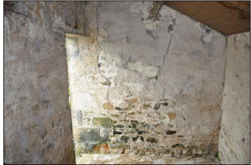
69. Internal view looking towards entrance
