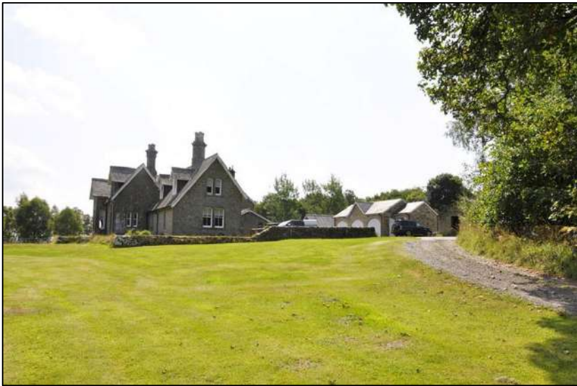
7. Looking south-east towards Evistones House and modern garaging
