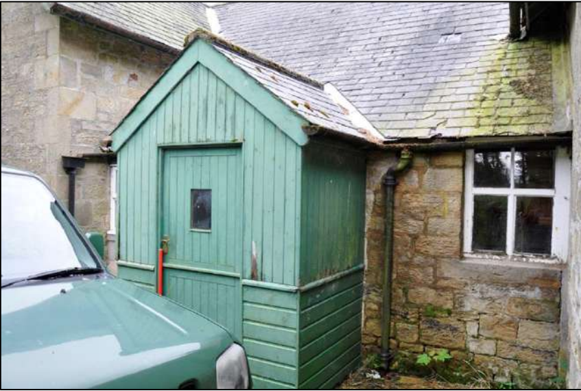
16. Kitchen and porch extension to north-west elevation
