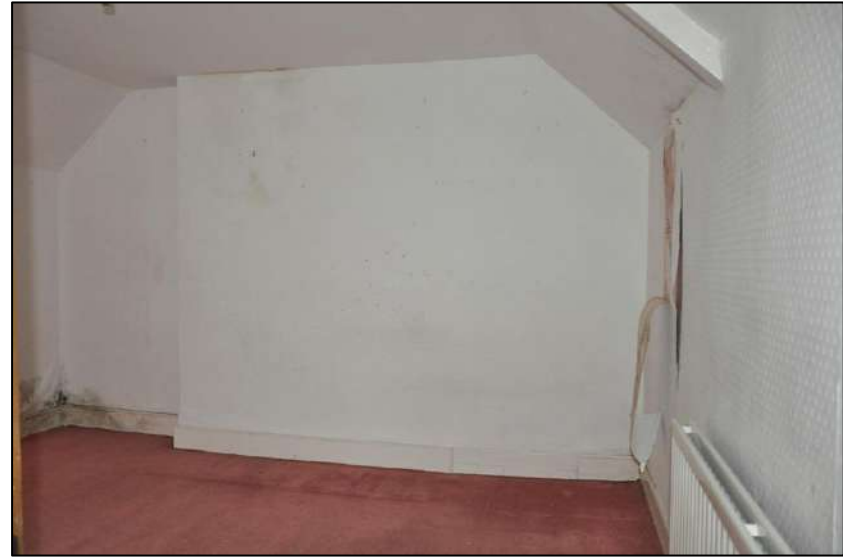
33. Fireplace removed and opening blocked, front (eastern) bedroom
