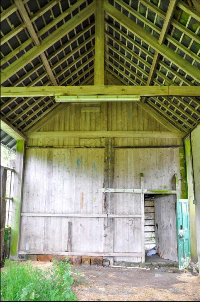
44. Modern hay barn with king post roof, looking towards timber partition to cart shed
