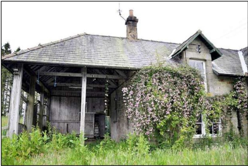
15. Hay barn (left) with dormer window over ground floor sashes to cottage, south elev
