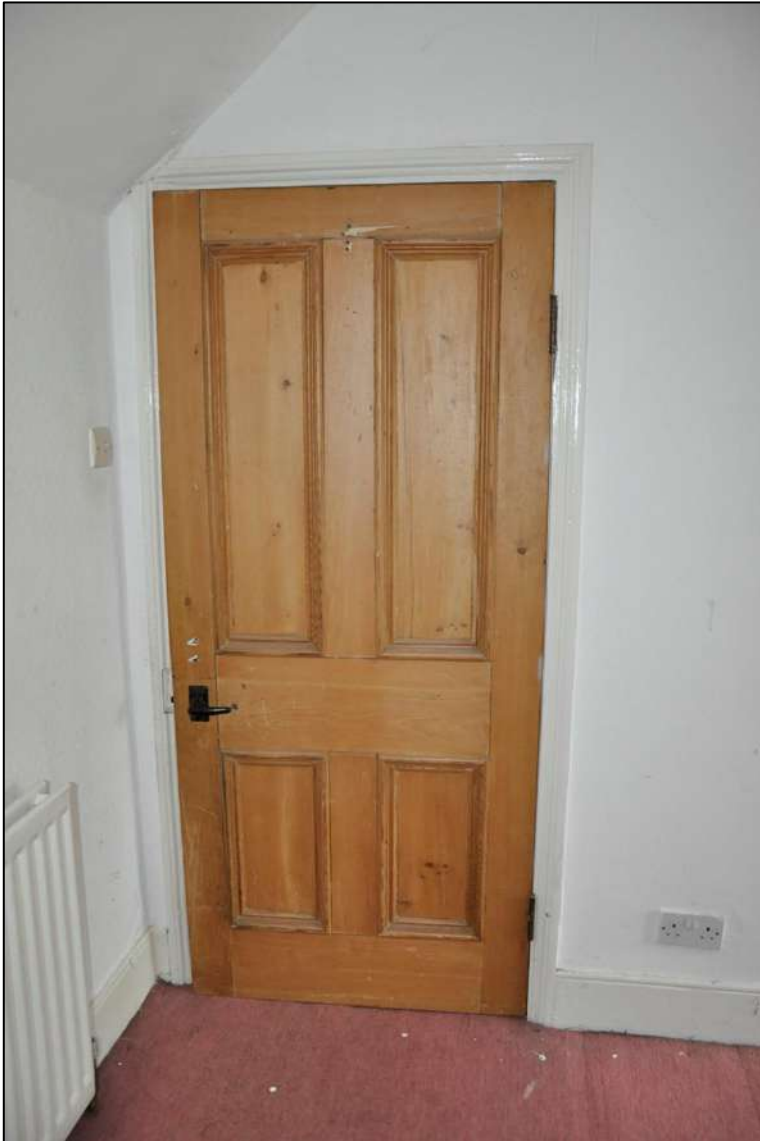
32. Original four-panel door set in moulded architrave, front (eastern) bedroom, first floor
