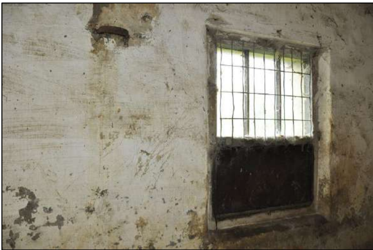
73. Detail of window viewed from inside kennel
