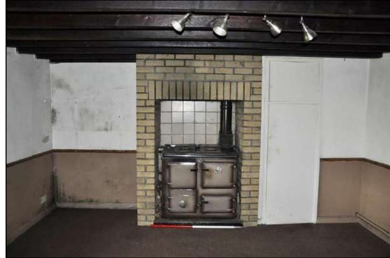
20. Rear parlour with exposed timber ceiling joists and 20 th century brickwork surround to Aga that has replaced the original chimneybreast and fireplace. 20 th century dado rail
