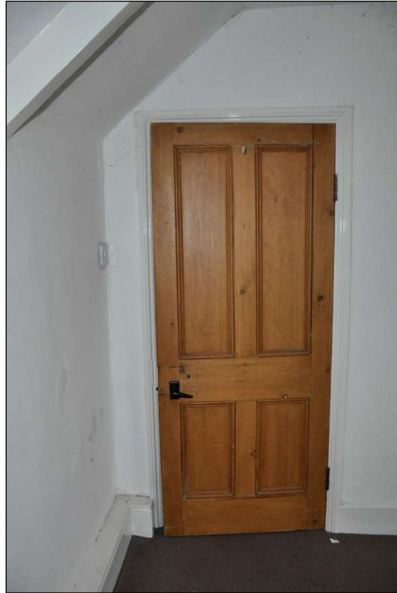
36. Original four-panel door set in moulded architrave, rear bedroom
