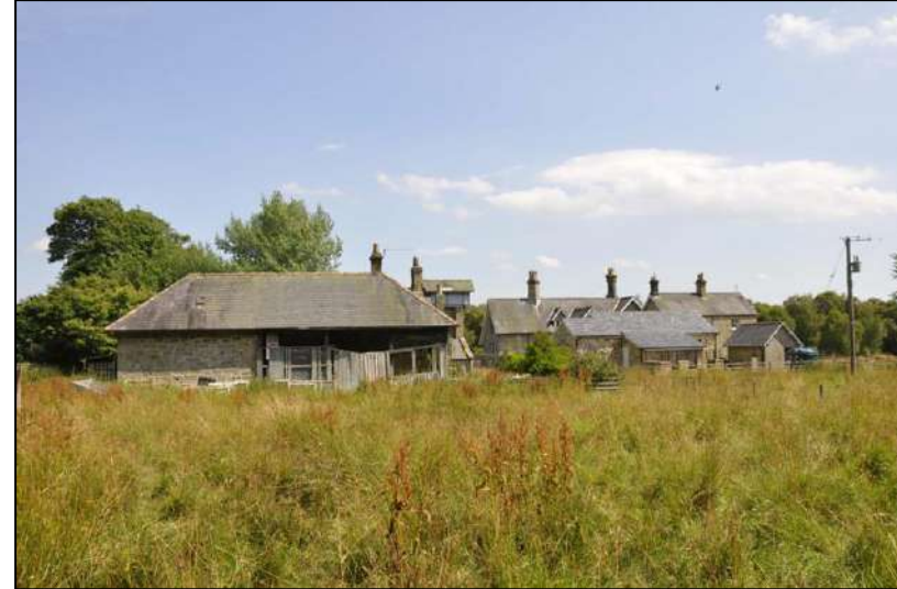
2. Looking north-east from field towards hay barn and cart shed (left) and modern kennels/garaging with Evistones House to rear (right)
