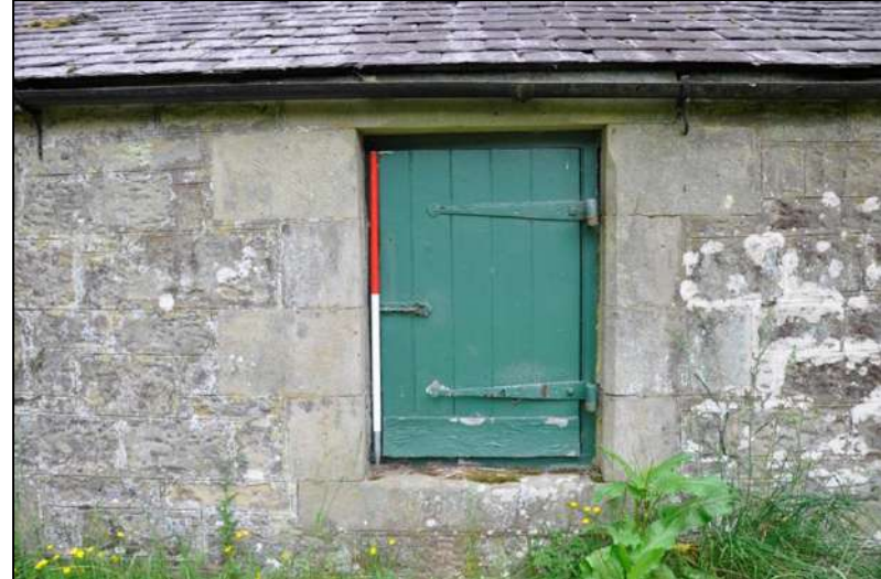
48. Stone surround to vertical boarded hatch door to store with strap hinges (1m scale)
