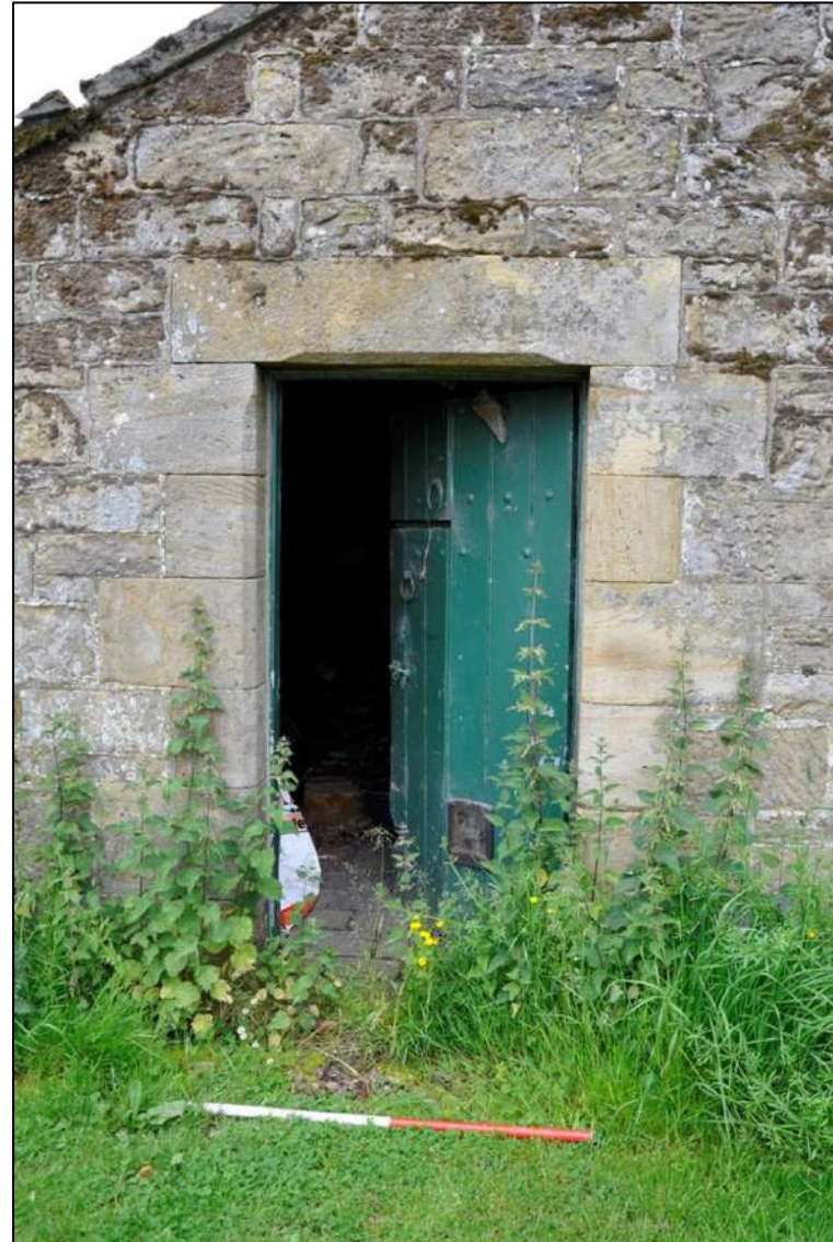
52. Detail of entrance to stable with centrally hinged vertical plank door with horseshoe denoting former function (1m scale)
