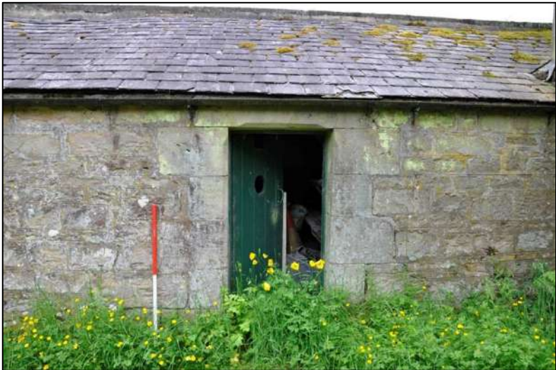
49. Stone surround and chamfered lintel to store (1m scale)
