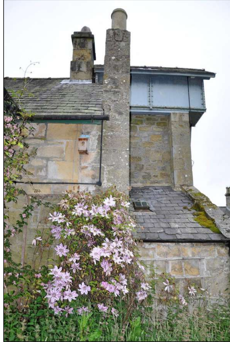
75. Quoins mark end of cottage with boiler house, chimney, water tank extension
