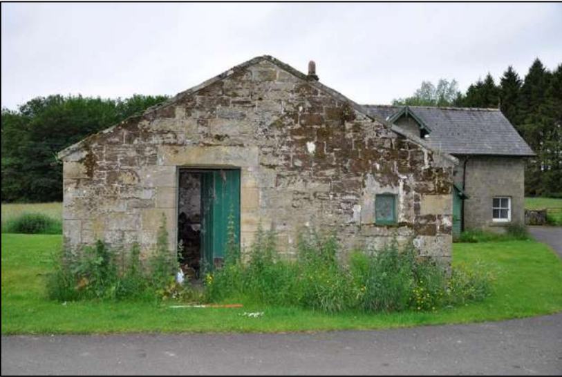
51. North gable end to stable with stone surrounds to entrance and small window
