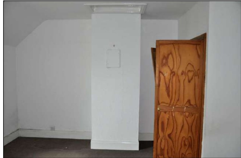
34. Chimneypiece, blocked fireplace, rear bedroom
