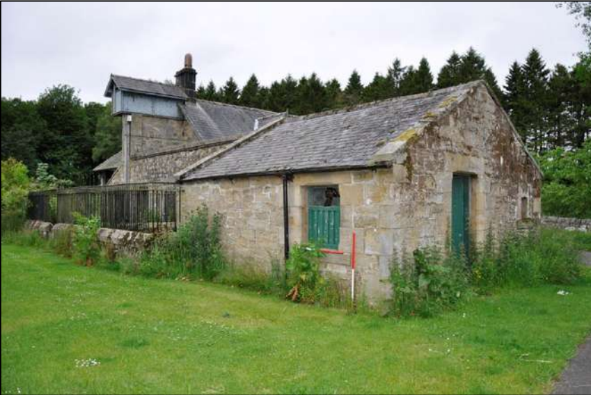
53. South-east elevation to stables with ventilated timber window (1m x 1m scale)
