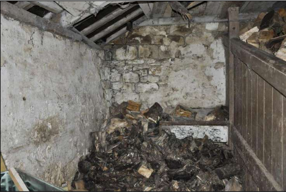
57. Trough against wall and central stall within stable. Lime render to walls
