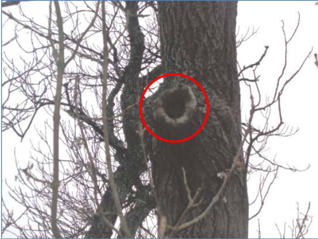
Photograph 9 – Potential bat roosting feature marked as TN3 in Appendix 2.
