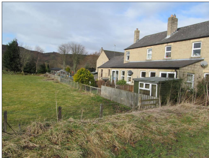
View looking towards proposed site from most recent houses on village outskirts [F]
