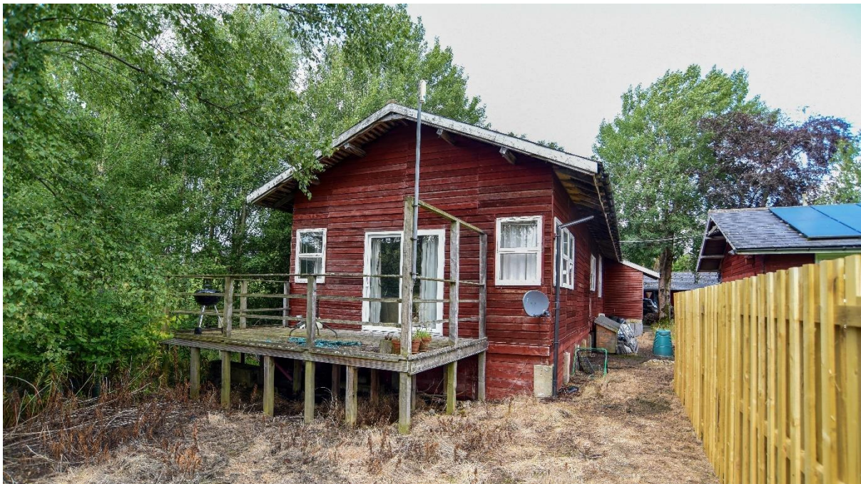
image b | Existing south elevation with deck and boundary fence to the right. Wansbeck house roofline is seen to the right
