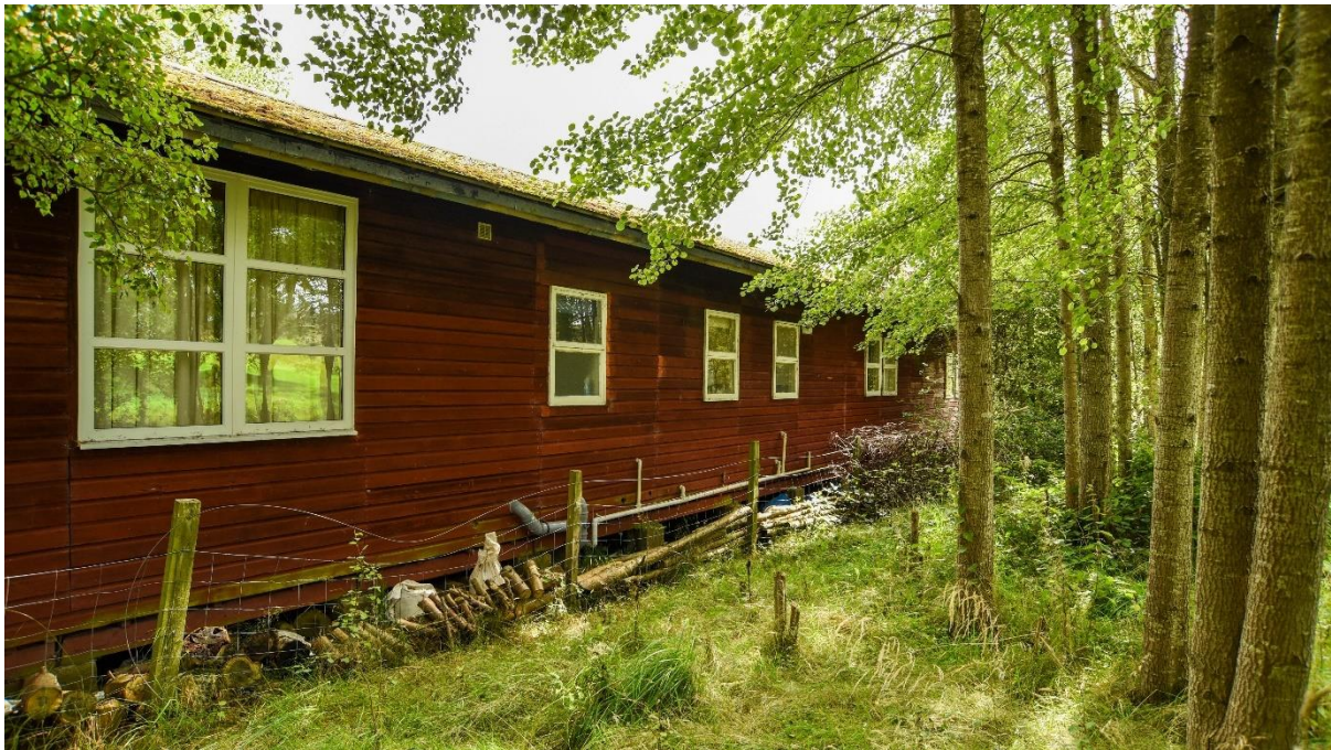
image c | West elevation, facing onto trees within the grounds of Brown Rigg Lodges. No changes are proposed to this elevation.
