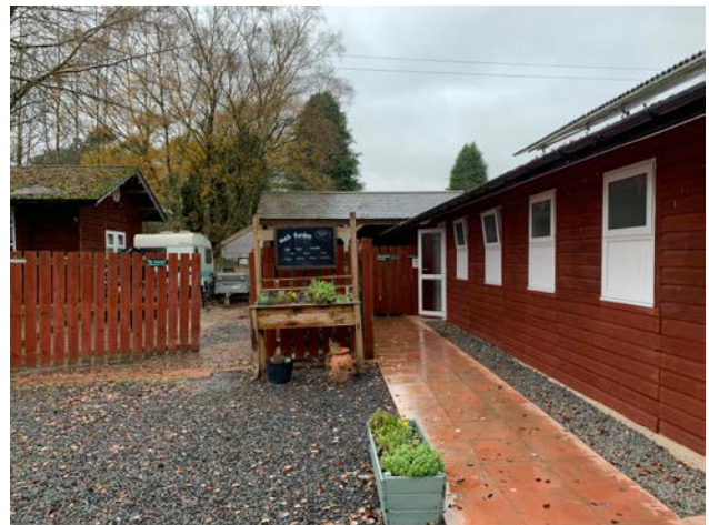
Fig 6 House to left and utility building to right
