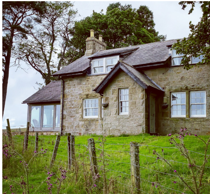
Fig 1. Existing photo of cottage
